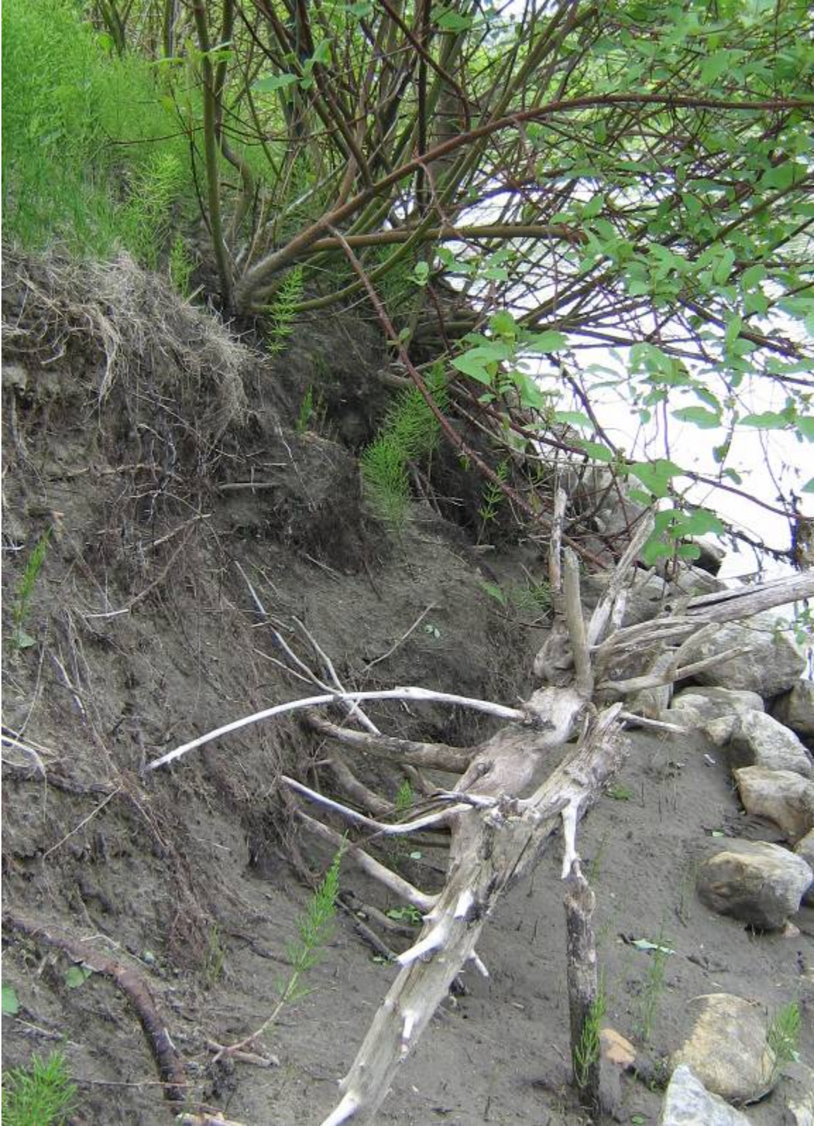
Photo 7 – Area 5: Example of near vertical face proposed for removal.
