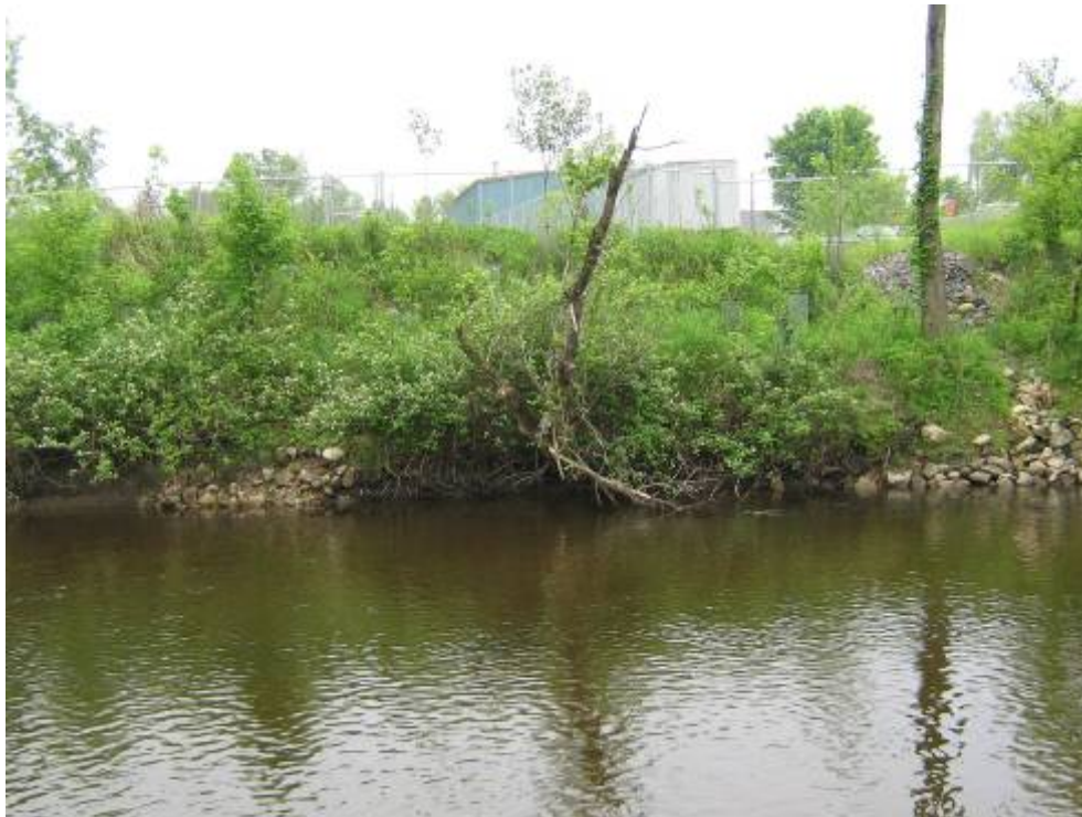
Photo 2 – Area 2: Approximately 40 feet of undercut bank upstream of swale.
