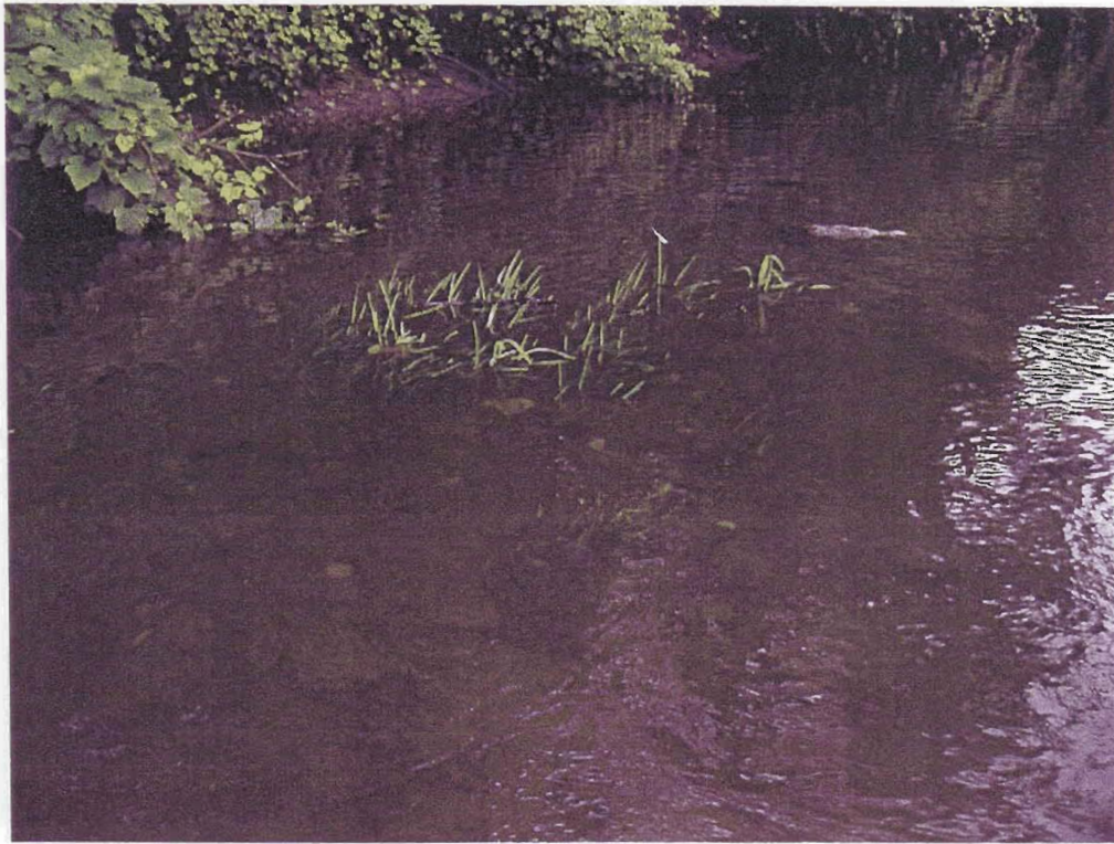
Photograph 1: Cell B, Vegetation growing in center of single wing deflector
