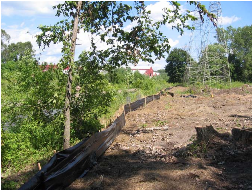
Photograph 6: August 2005; Planting Area 16 showing impacts of ongoing remedial action work
