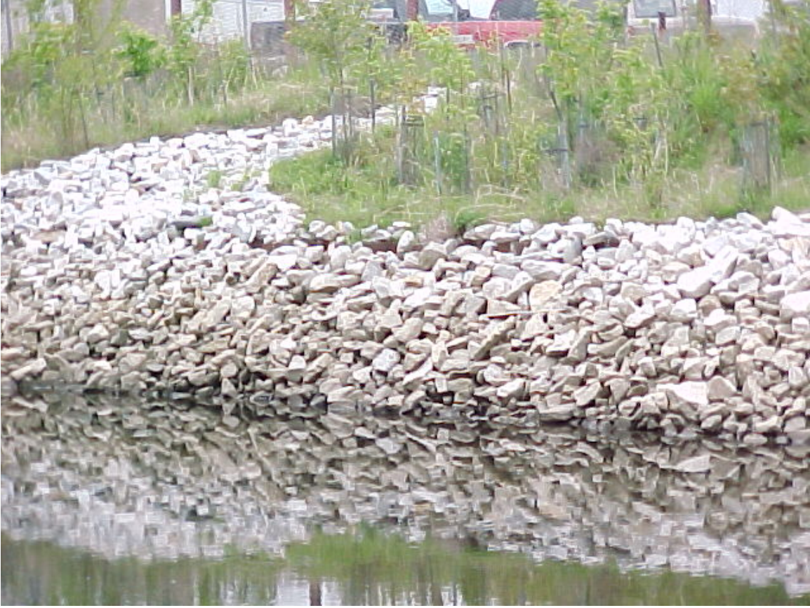
Photo 3 – Area 2: Exposed sheetpile tops.
