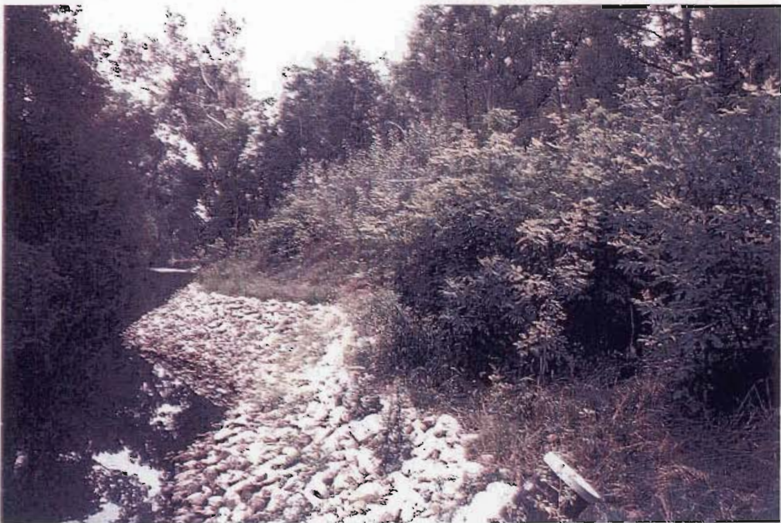
Photograph 4 Planting Area 2, Viewed Looking Downstream
