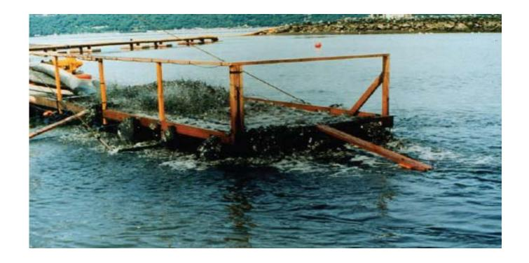
Pilot study cap material placement anticipated to be completed using a spray and/or spreader box application of a slurry of isolation layer material and lake water.
