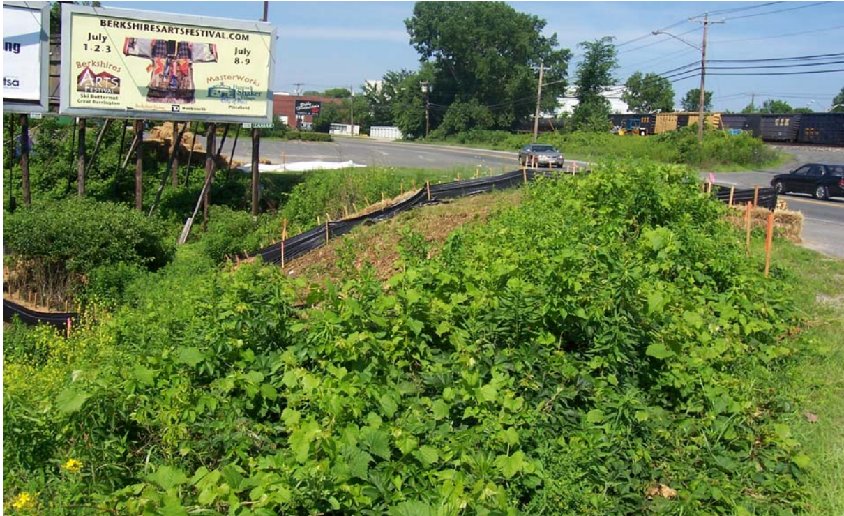
Photo #1: Site preparation and installation of silt fencing and hay bales.
