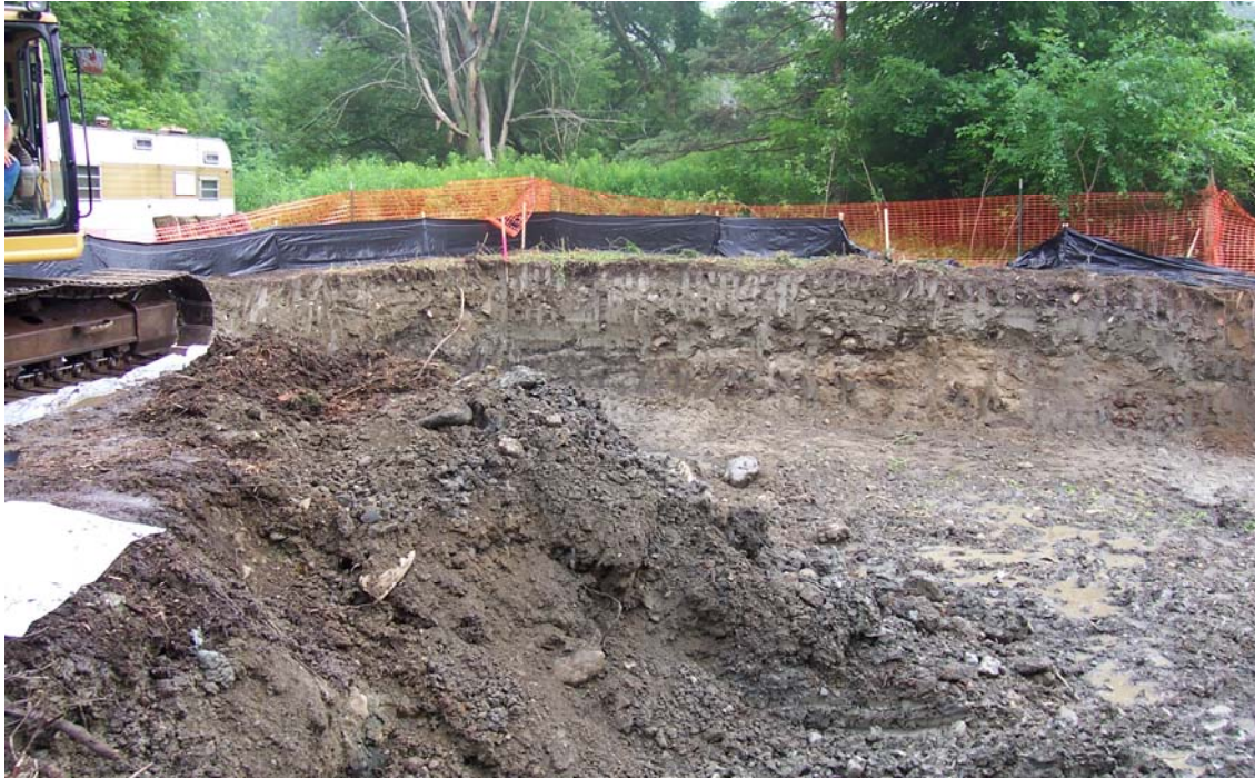
Photo #5: Performance of removal activities.
