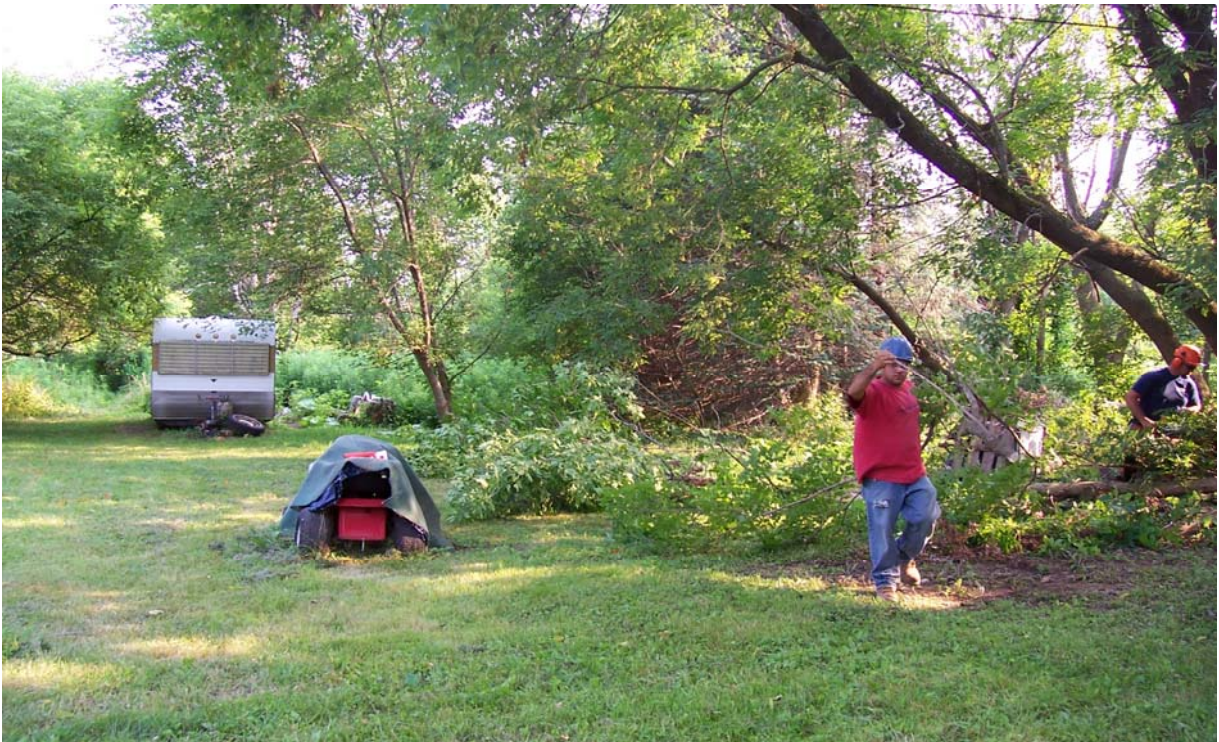
Photo #4: Clearing of vegetation in preparation for removal activities.
