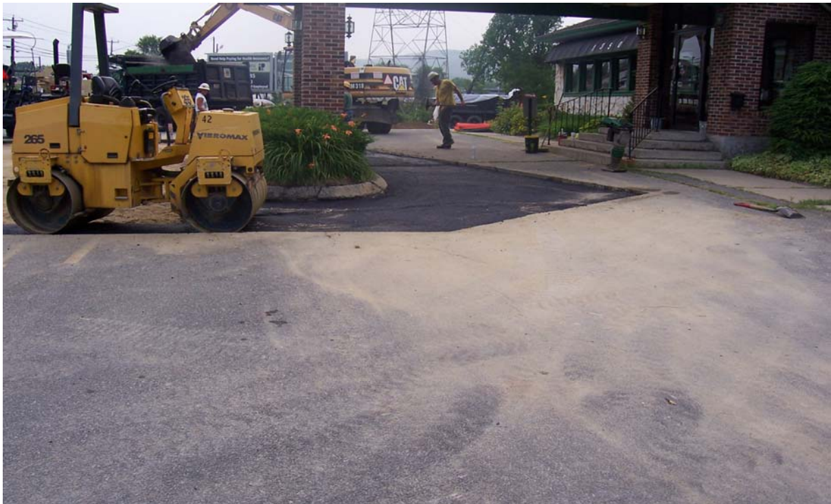
Photo #8: Restoration of asphalt surfaces.
