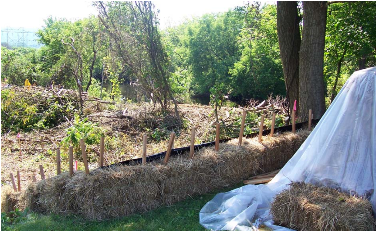
Photo #2: Site preparation and installation of silt fencing and hay bales.
