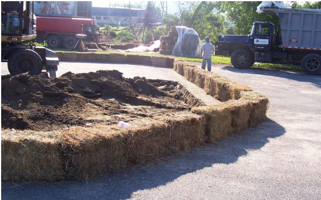
Photo #6: Performance of removal activities.
