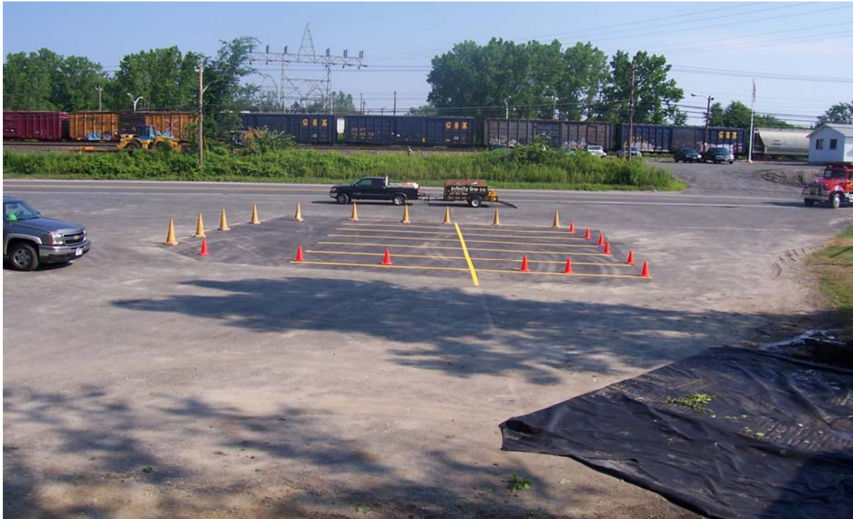
Photo #9: Completed restoration of asphalt surface.
