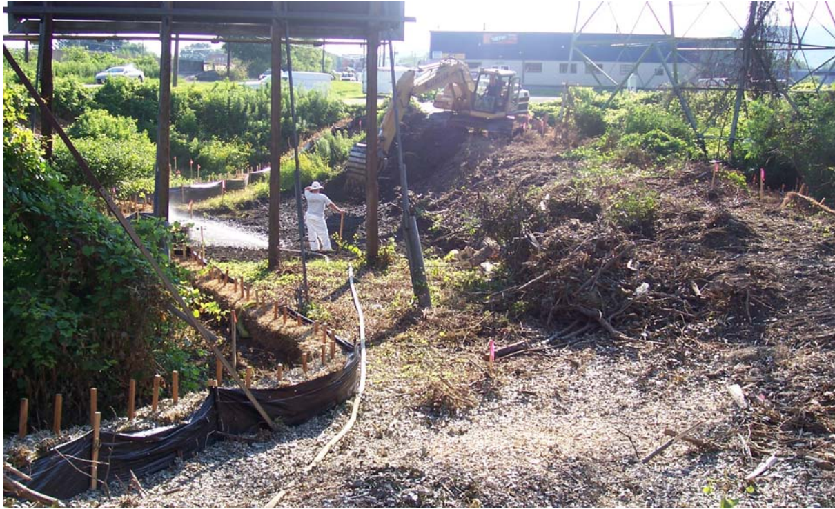
Photo #7: Performance of soil removal activities.
