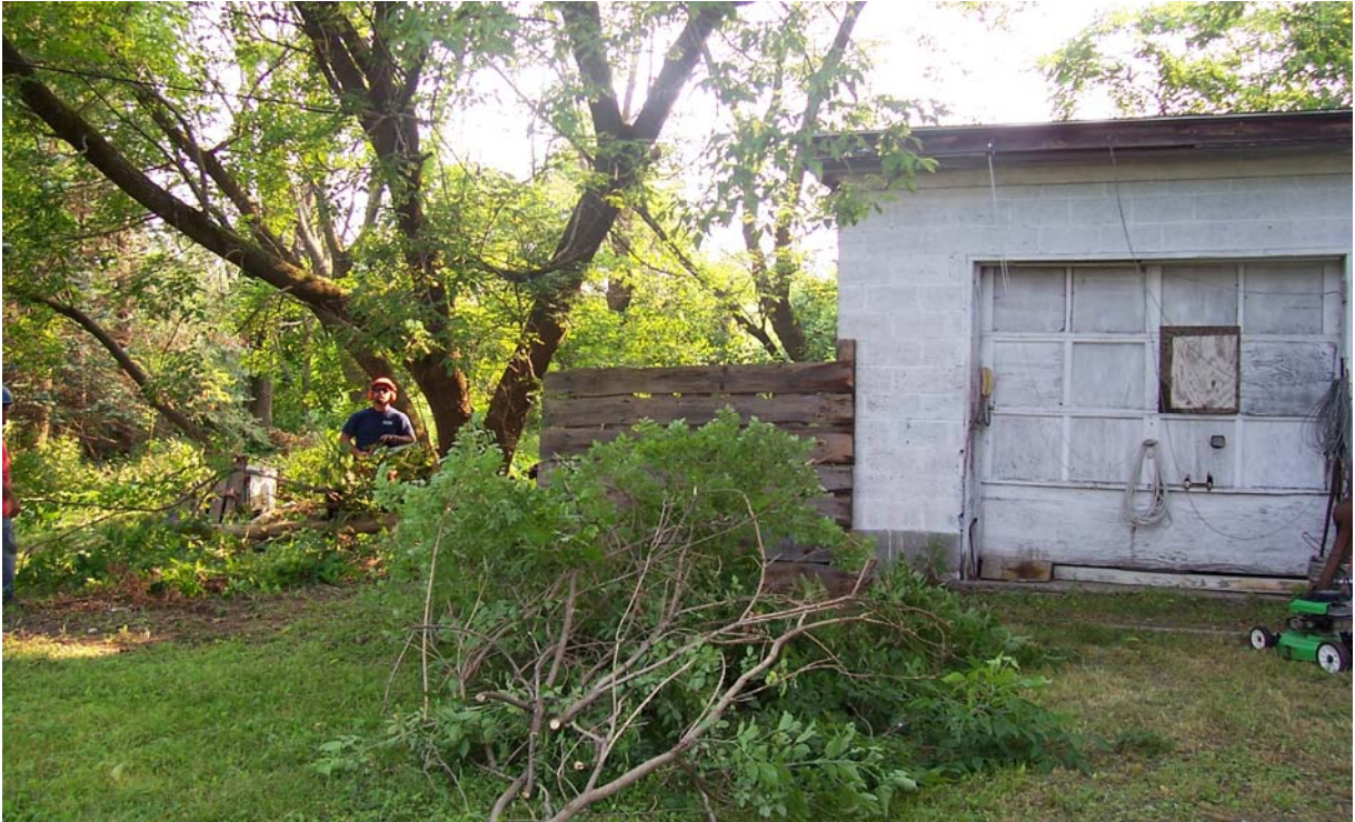
Photo #3: Clearing of vegetation in preparation for removal activities.
