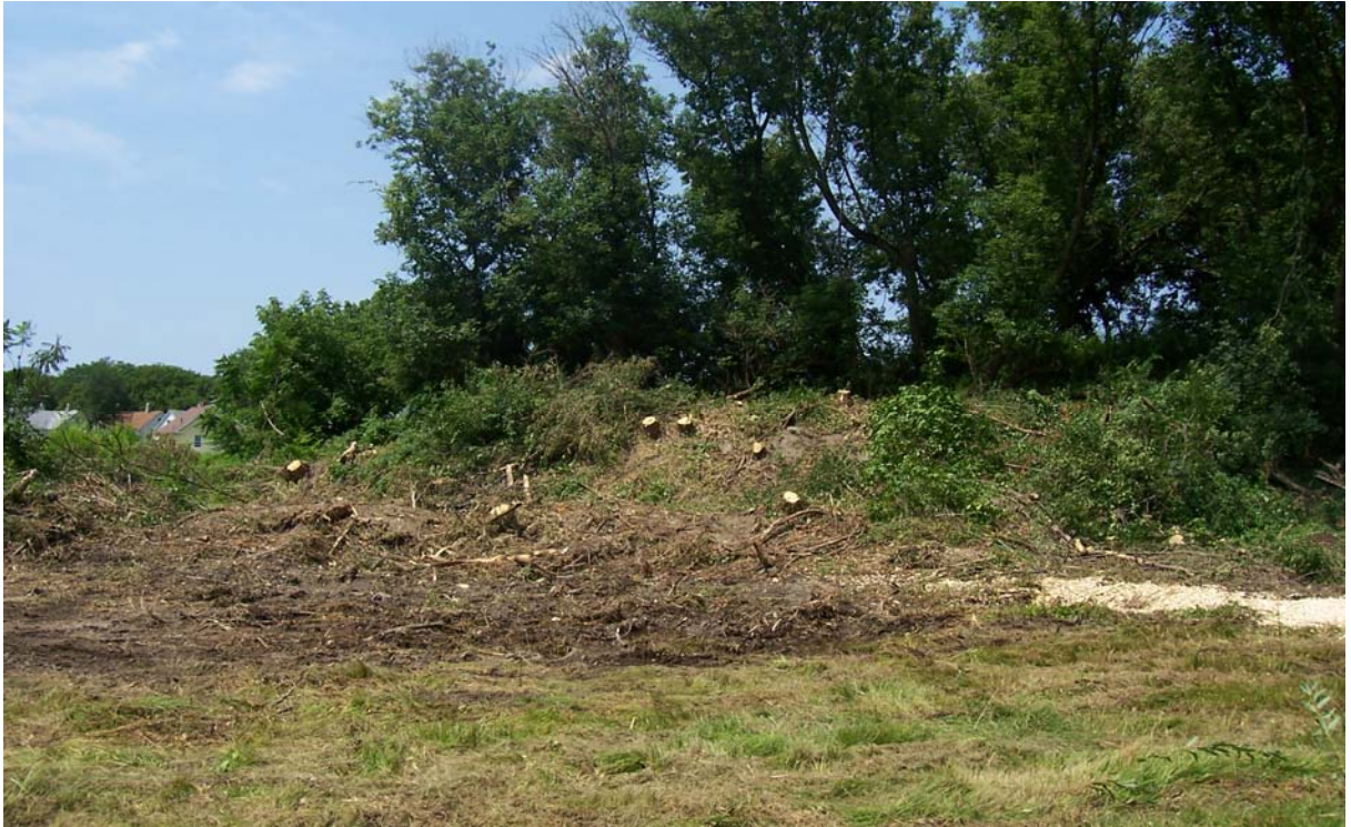
Photo #1: Clearing of vegetation in the vicinity of soil pile.
