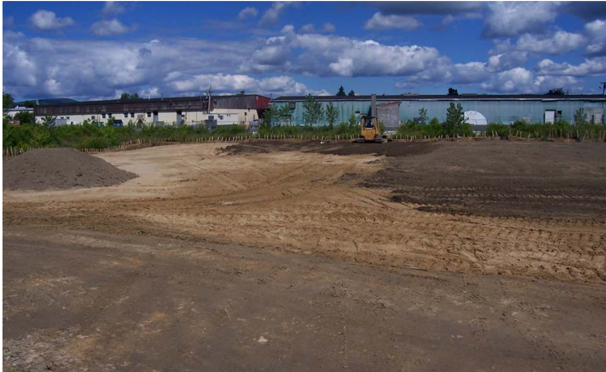
Photo #10: Backfilling and grading of excavations.
