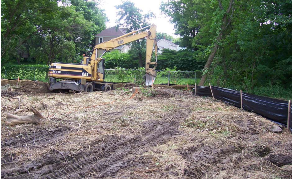
Photo #5: Performance of soil removal activities.
