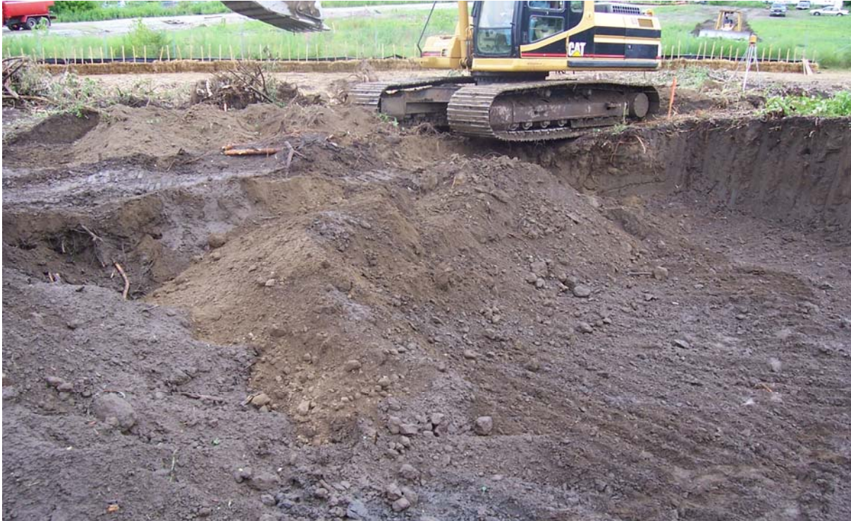
Photo #3: Performance of soil removal activities.
