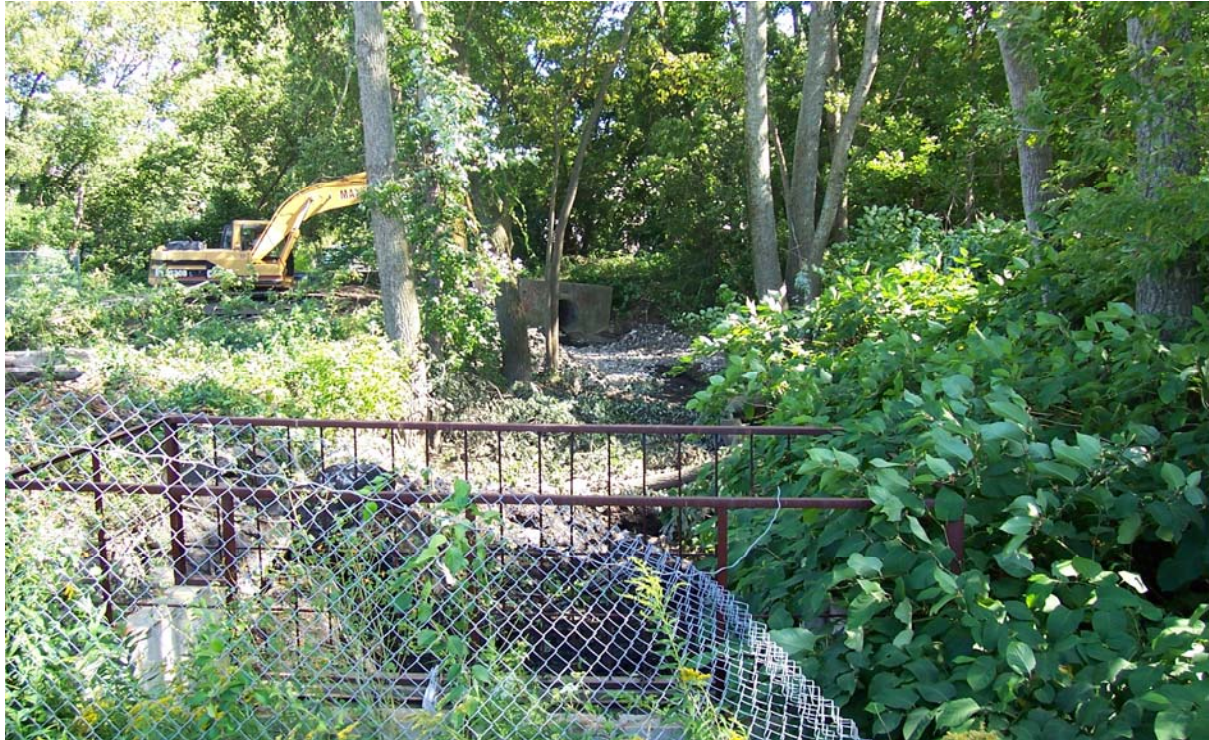
Photo #15: Restoration of drainage swale in vicinity of Day Street.
