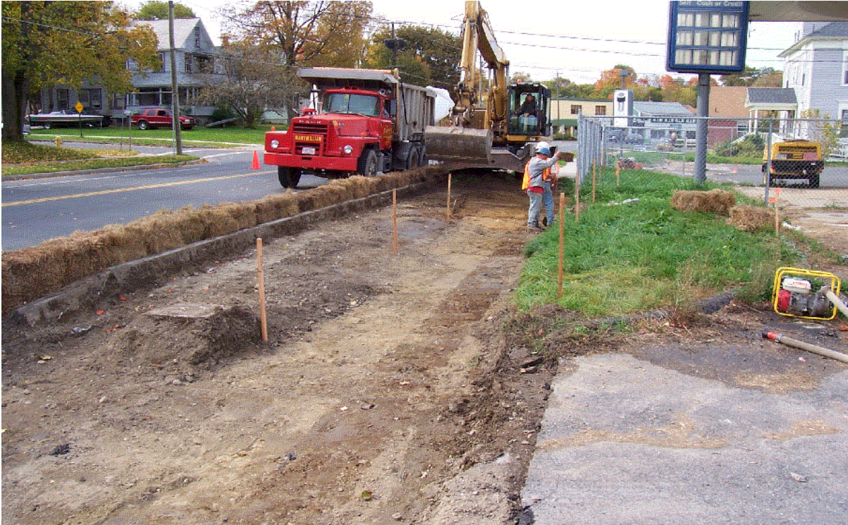
Photo #9: Completed excavation in vicinity of Parcels I8-23-4 and I8-23-5.
