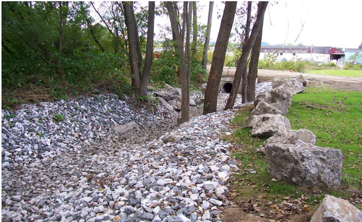
Photo #16: Restored drainage swale in vicinity of Day Street.
