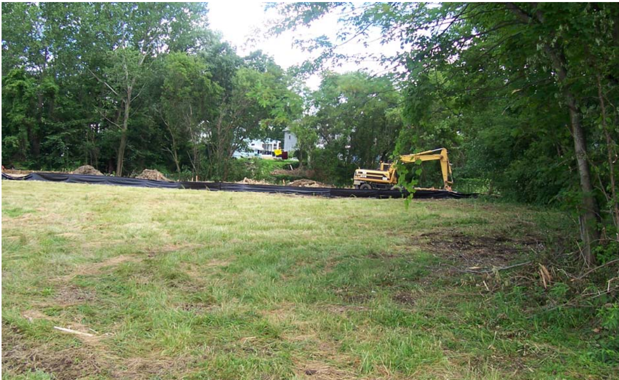
Photo #4: Performance of soil removal activities.
