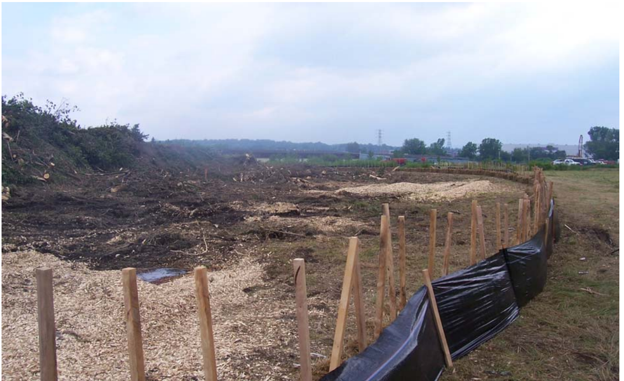
Photo #2: Site preparation in the vicinity of soil pile.
