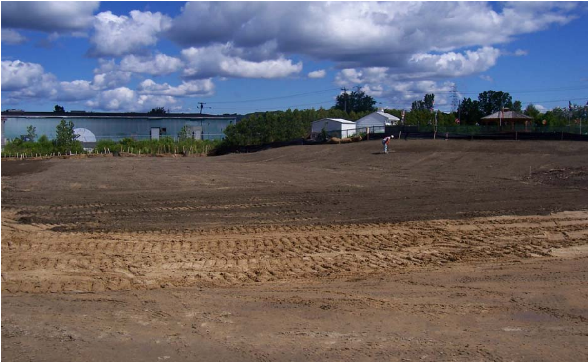
Photo #11: Performance of restoration activities.
