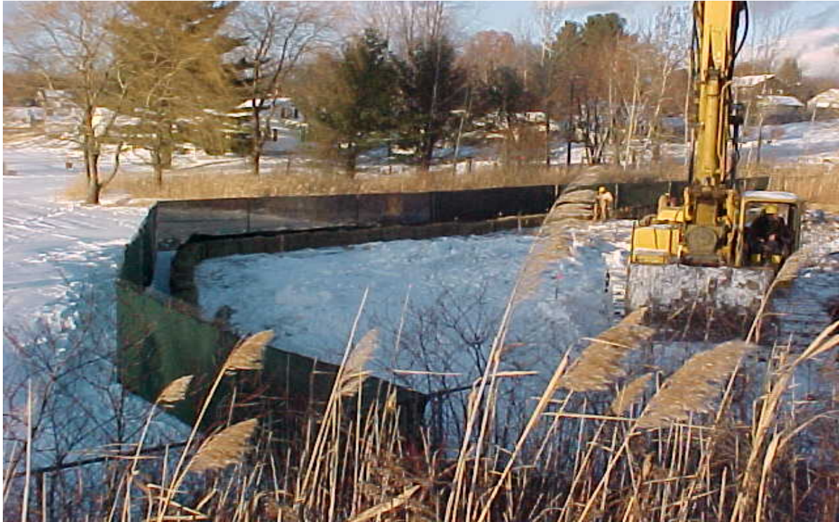
Photo #3: Initiation of excavation activities inside the excavation area.
