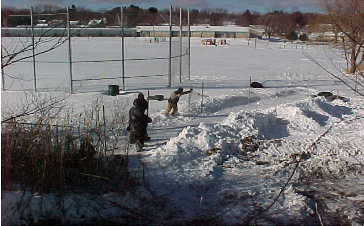
Photo #1: Installation of fencing around the perimeter of the excavation area.
