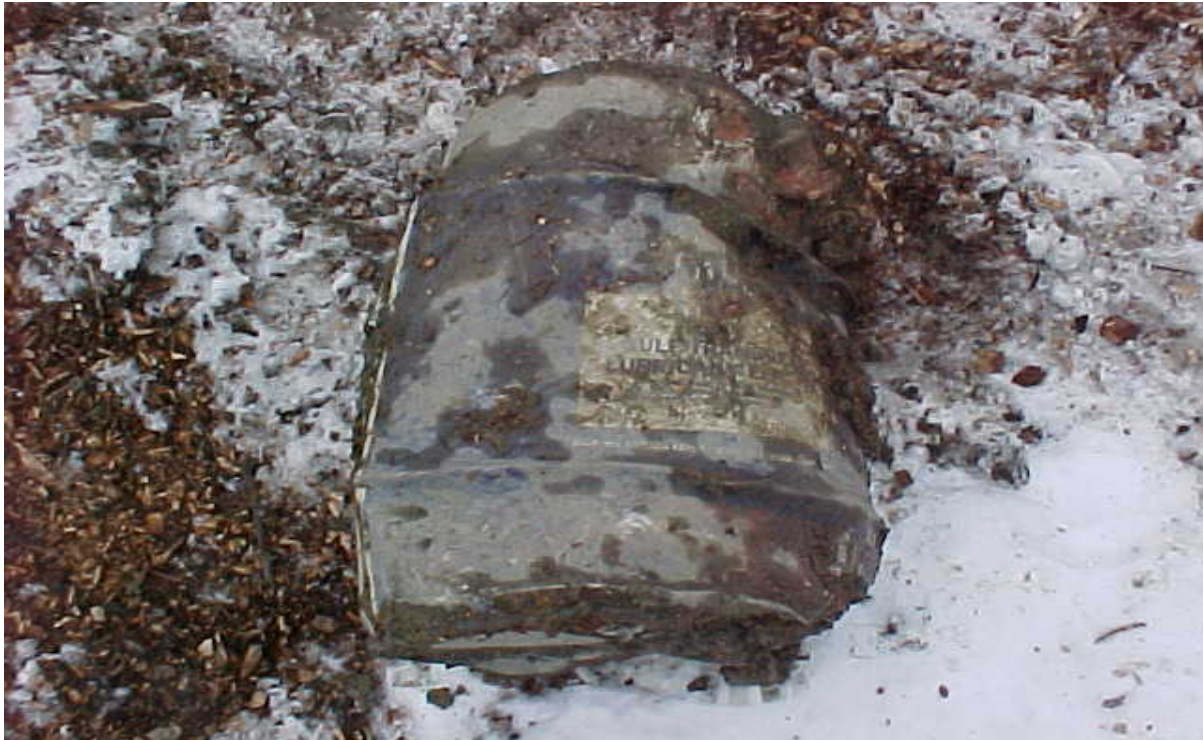
Photo #5: Photo of drum uncovered during excavation activities inside the removal area.
