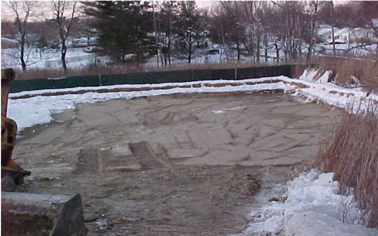
Photo #9: Photo of backfilled removal area.
