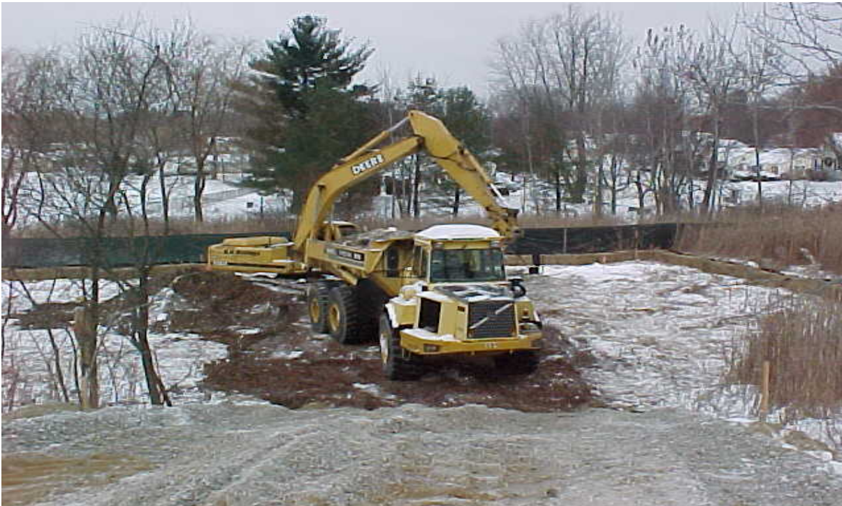
Photo #2: View of ramp constructed to access removal area.
