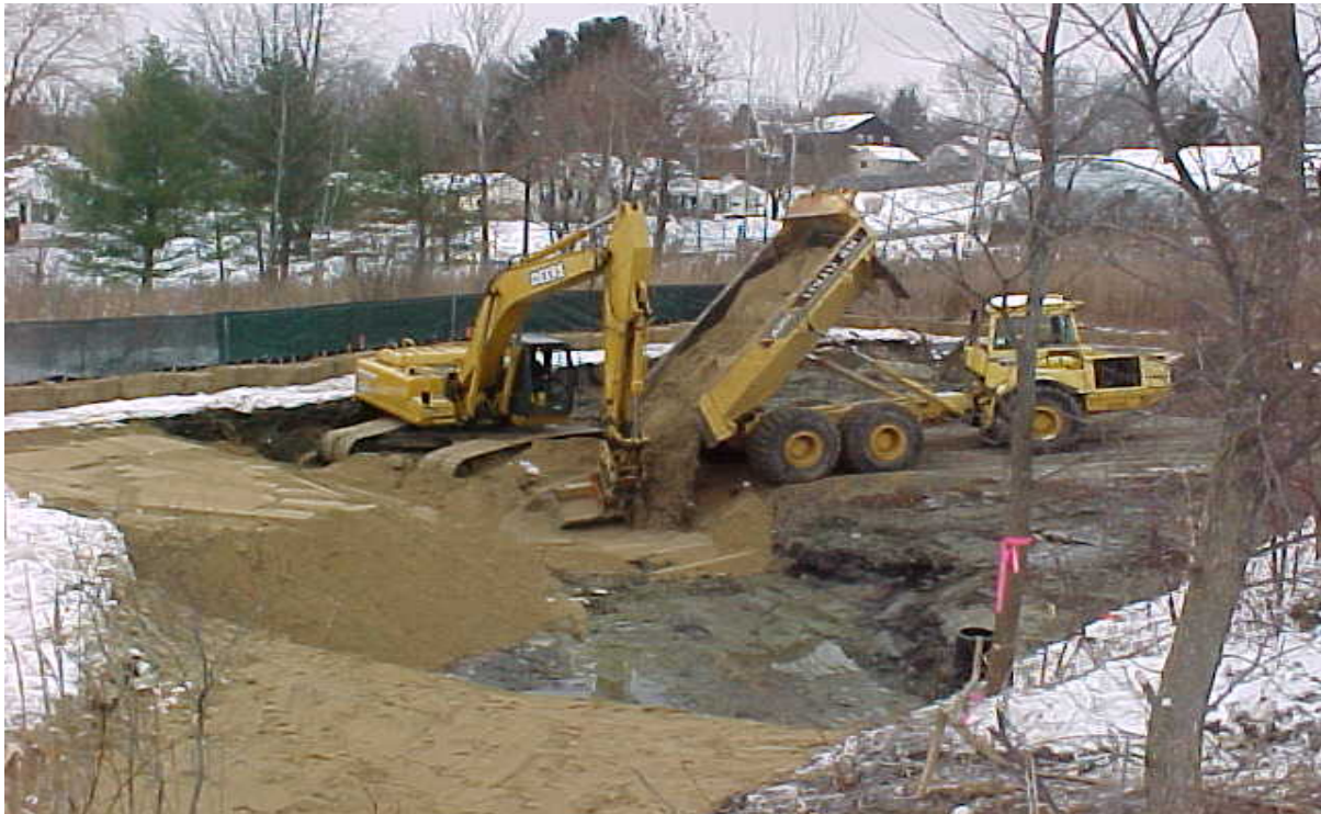
Photo #8: Backfilling activities inside the removal area.
