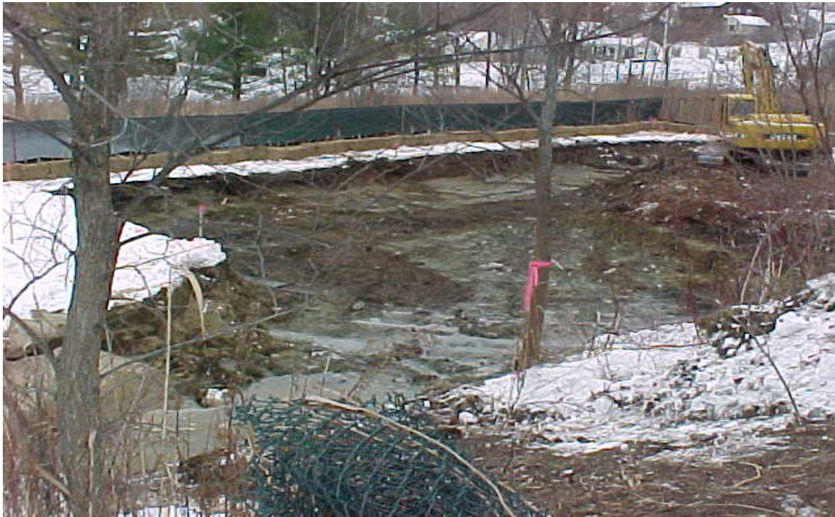
Photo #4: View of initial excavation activities inside the removal area.
