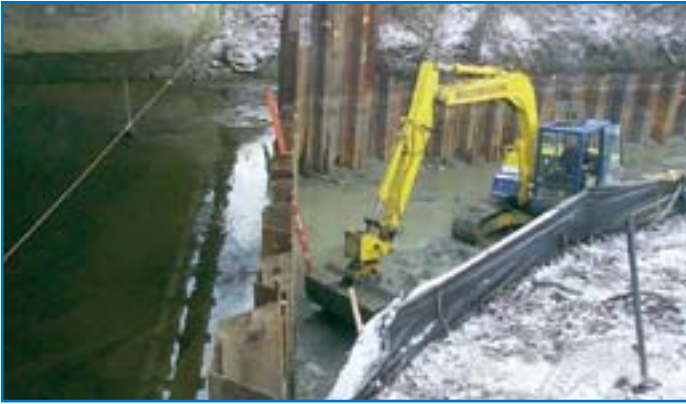
Excavation in Progress Within Typical Sheetpile Cell
