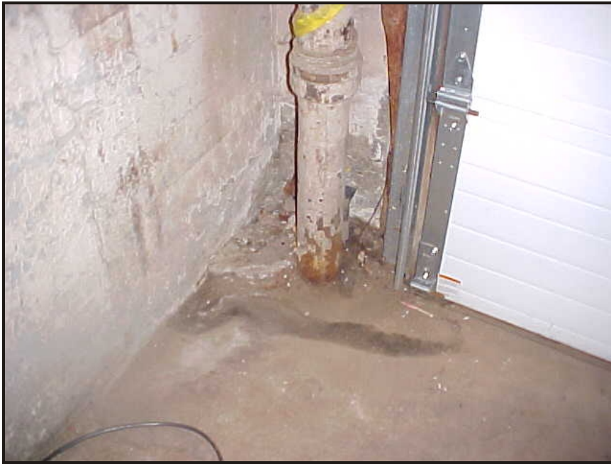
(3) Photo of a roof drain next to an overhead door just north of the new boiler room in an alleyway
