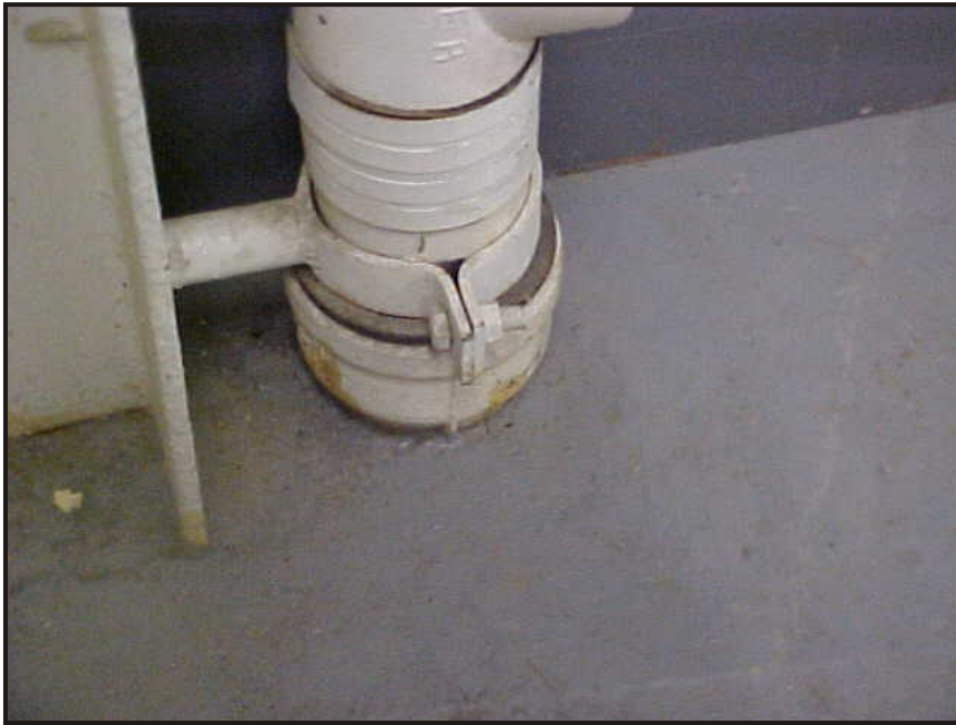
(9) Photo of a roof drain in the center of the mechanical room
