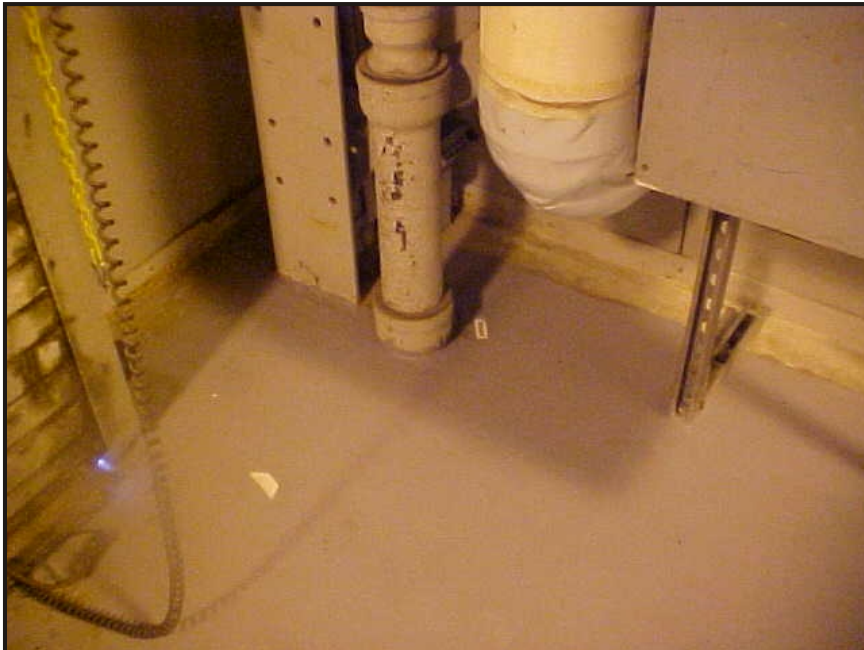
(22) Photo of a roof drain in the northeast corner of the loading dock area
