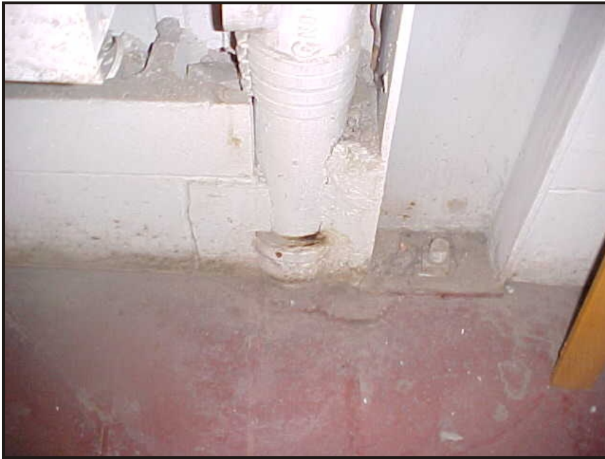
(15) Photo of a roof drain on the south wall of the record storage area room
