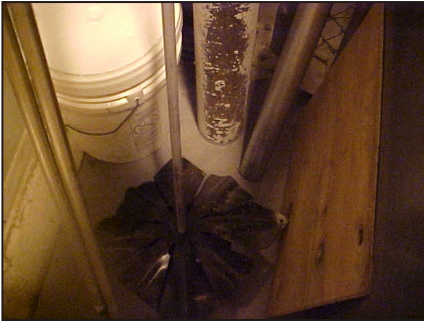
(21) Photo of a roof drain on the east wall of the maintenance shop
