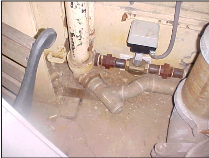
(15) Photo of a roof drain in the high bay storage area at the northwest corner of the building
