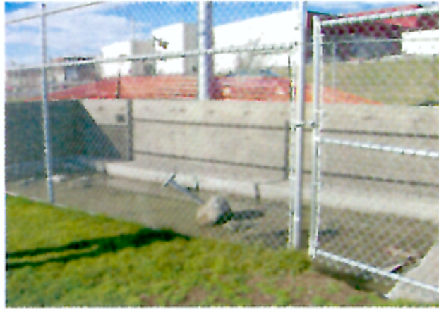
Photo #1: 3rd Base Dugout. Partial Concrete Slab/Wall Installation (11/18/05)
