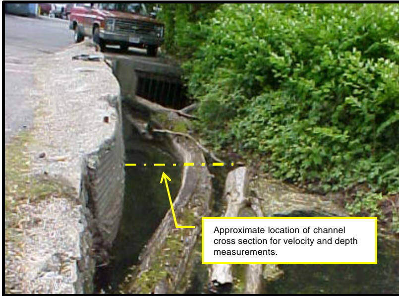
Outfall C: Looking downstream at channel and culvert to Housatonic River .
