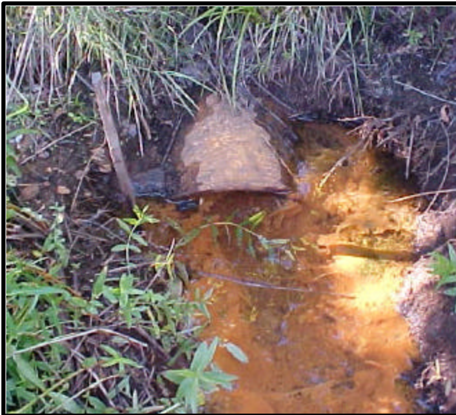
Outfall B: Showing conveyance after removal of sediment and debris.
