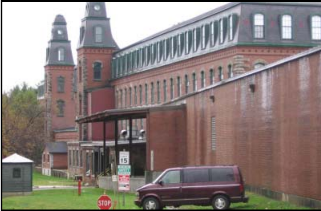
Figure 54. Rising Paper Mill, Housatonic, View South.
