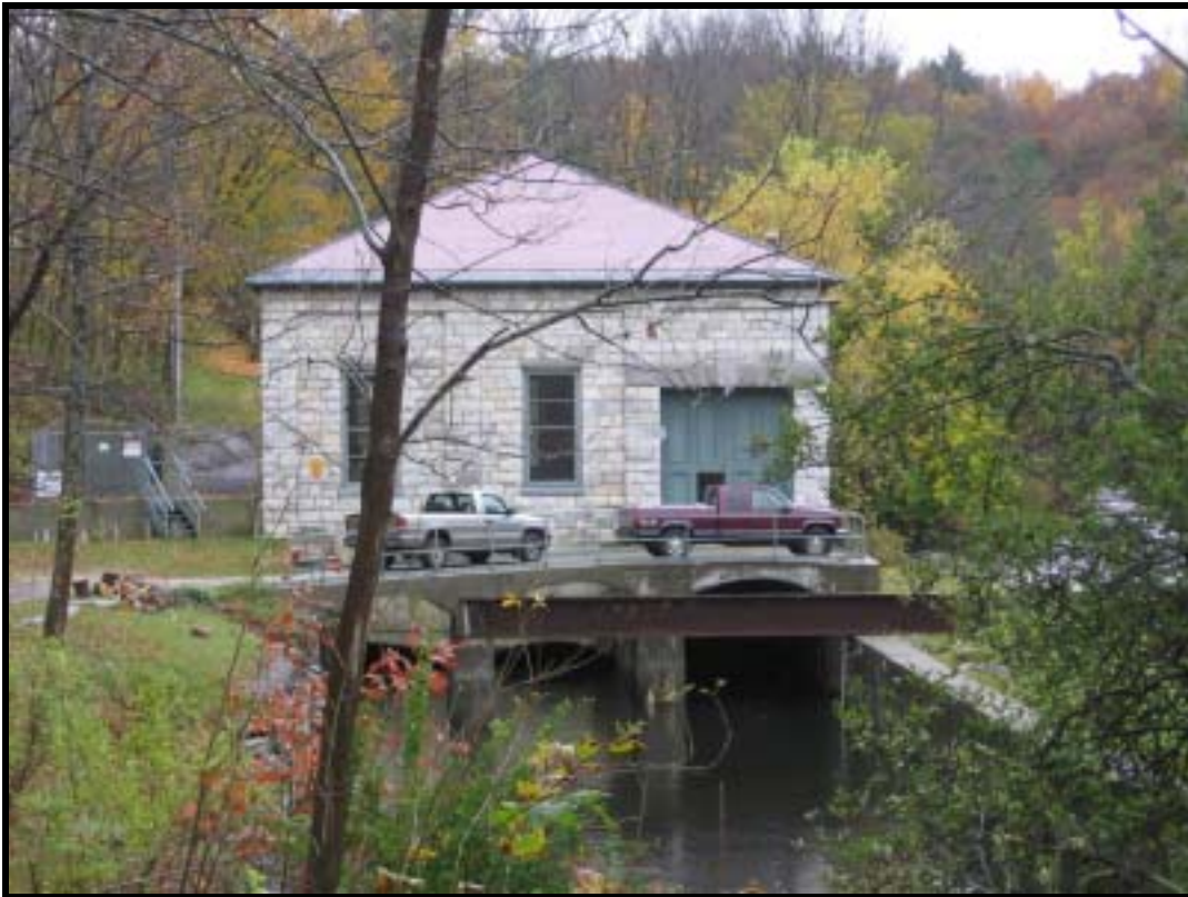
Figure 52. Glendale Power Station, Glendale, View Southeast.
