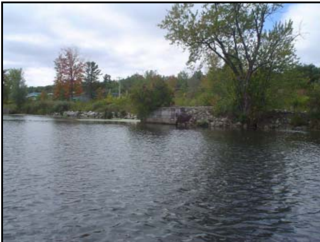
Figure 40. Dam/Bridge Remnants Just North of Current Woods Pond Dam, View West.
