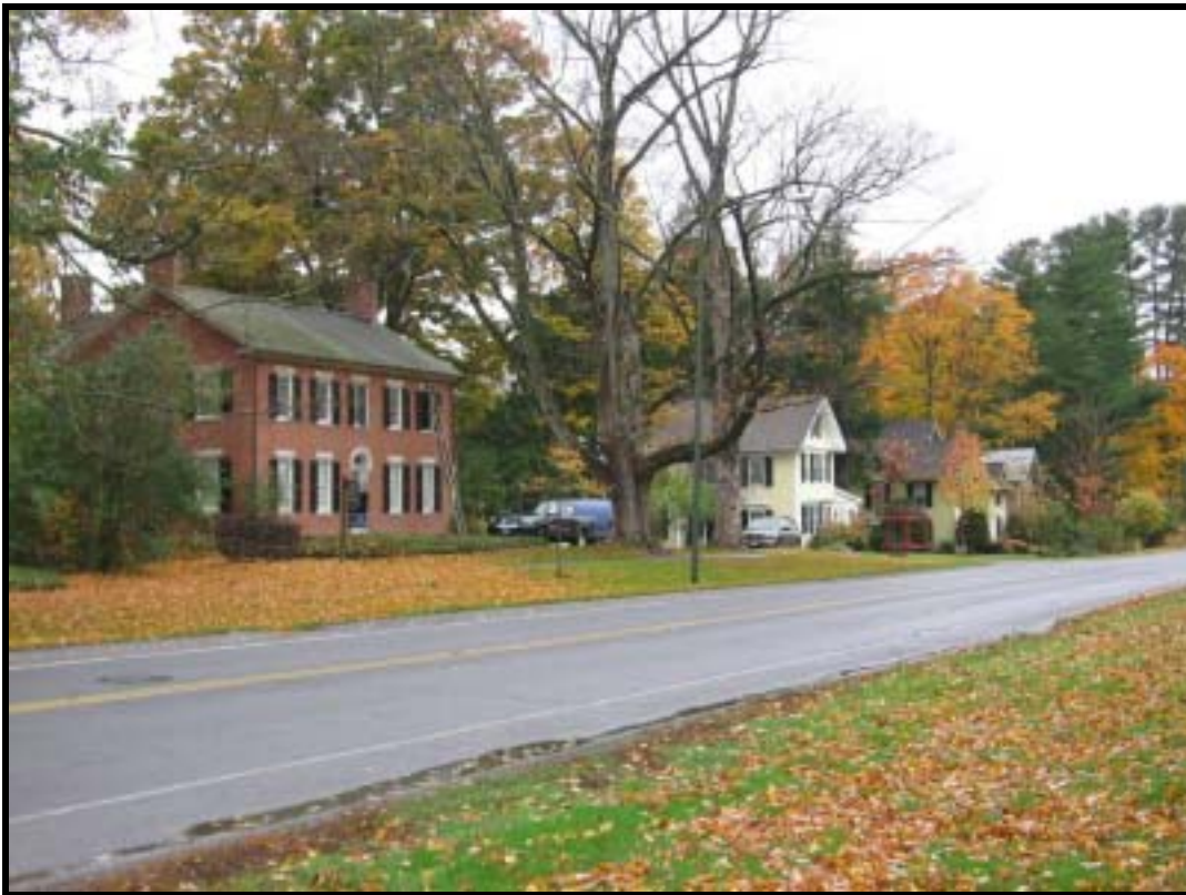
Figure 50. Streetscape, Main Street, Stockbridge, View West.
