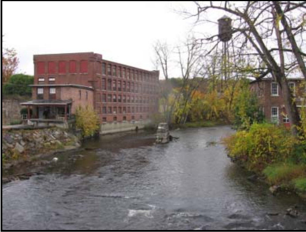
Figure 53. Monument Mills, Housatonic, View North from Route 183 Bridge.
