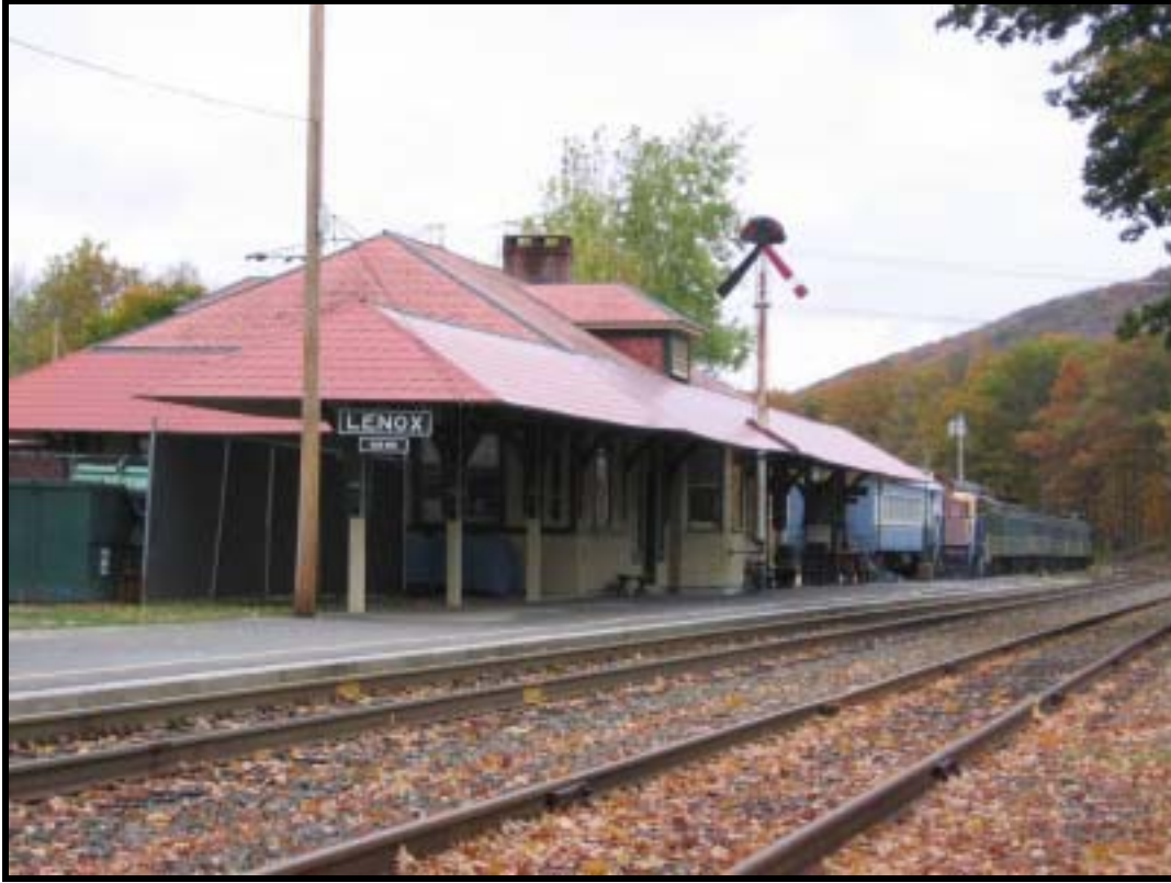
Figure 41. Train Depot, Lenox Station, View North.
