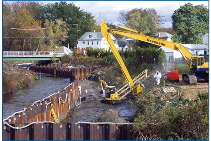
Removal – Excavation in the “Dry”
