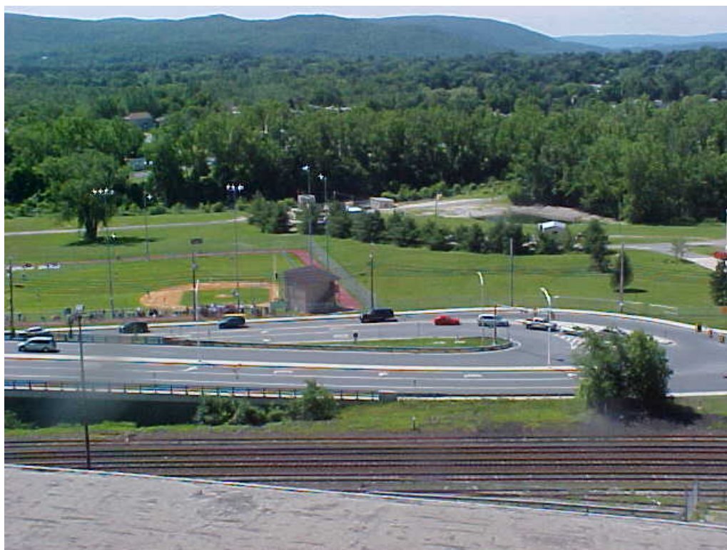
Photograph 23 Ballfield Area following completion of restoration activities. Photo taken looking southwest.
