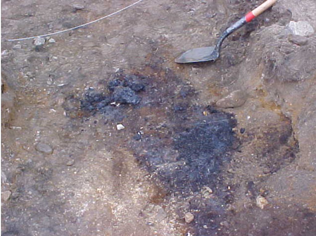
Photograph 6 Stained soil uncovered at the northeast corner of the scorer's booth during excavation for the footer.
