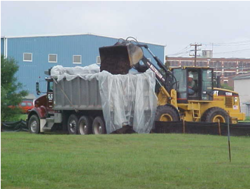
Photograph 12 Contractor loading soil into poly-lined trucks. Photo taken looking west.
