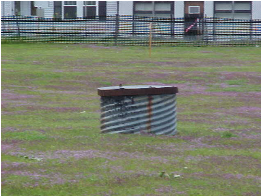
Photograph 2 36-inch diameter metal caisson located along the southern edge of the CRA to be removed. Photo taken looking east.
