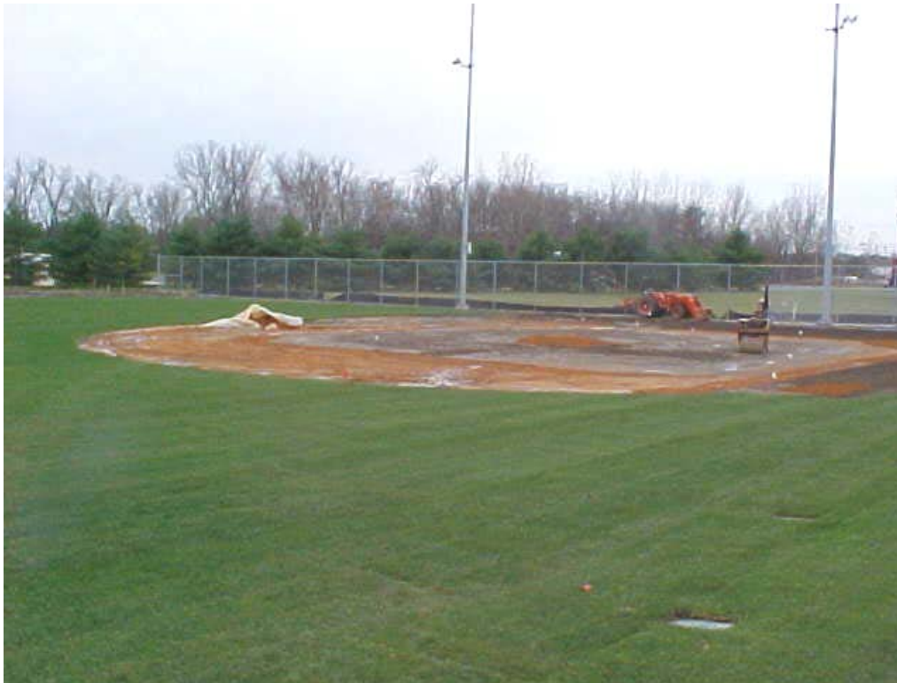
Photograph 20 Baseball field during placement of infield clay. Photo taken looking southwest
