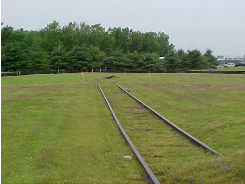
Photograph 1 CRA prior to initiation of work. Stakes from existing conditions survey and silt fence are visible in the background. Existing rail lines are visible in the foreground. Photo taken looking west.
