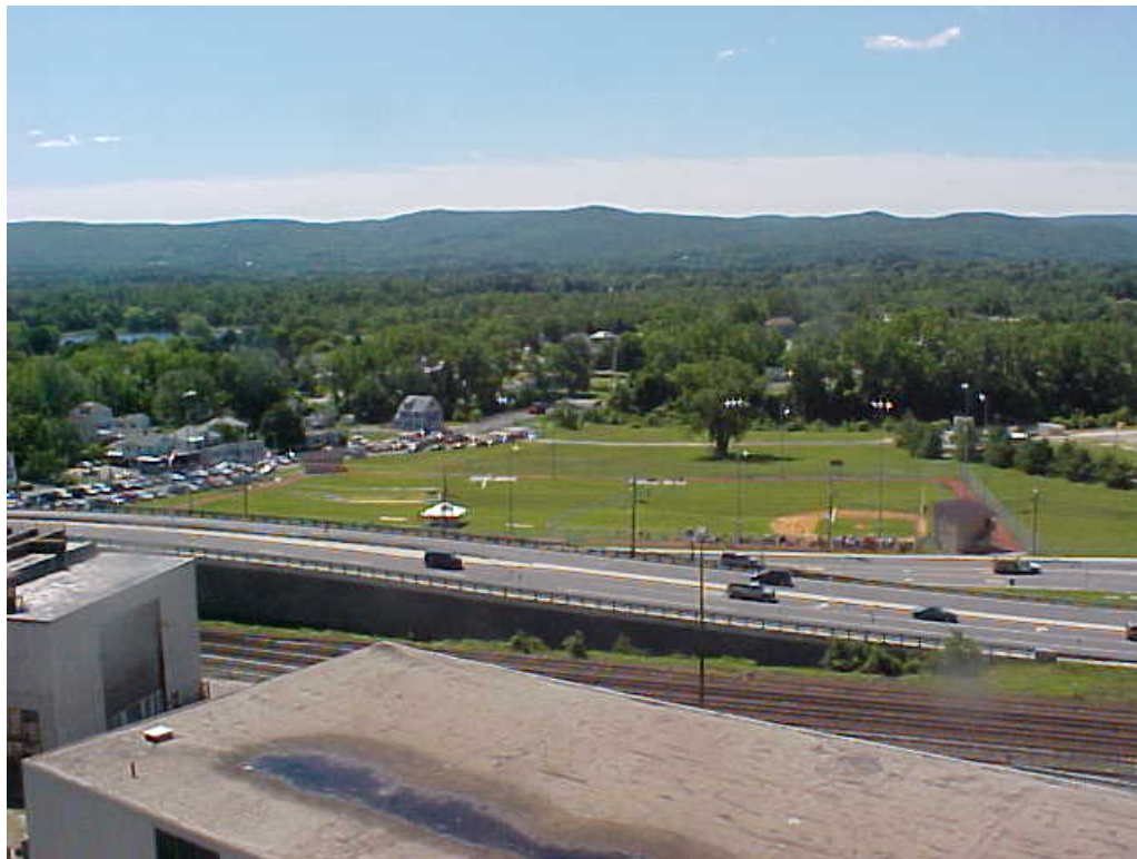
Photograph 22 Ballfield Area following completion of restoration activities. Photo taken looking south.
