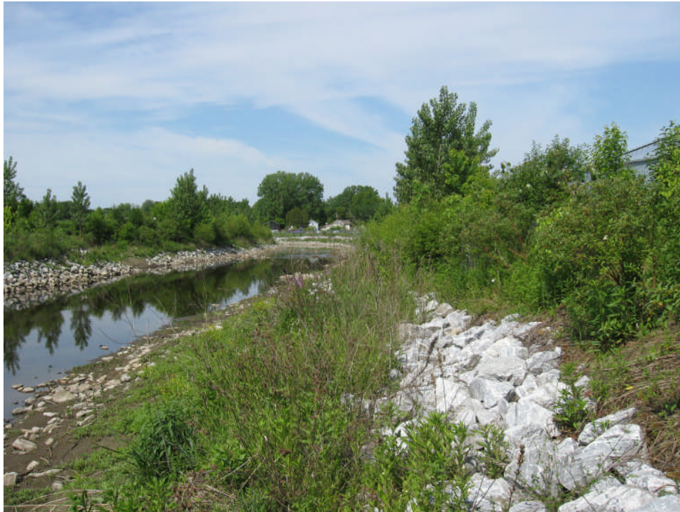
Photo 3: Monitoring Plot 1-W-1, facing downstream (to the southwest).
