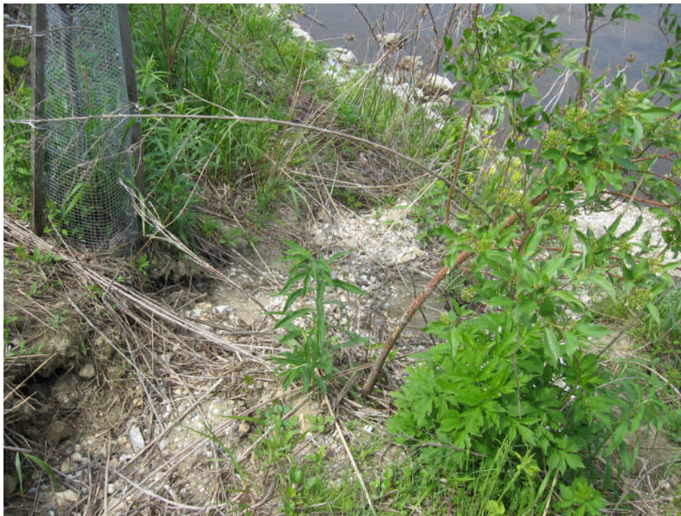
Photo 18: Alternate view of erosional swale within Planting Area #5, facing down-slope towards the river.
