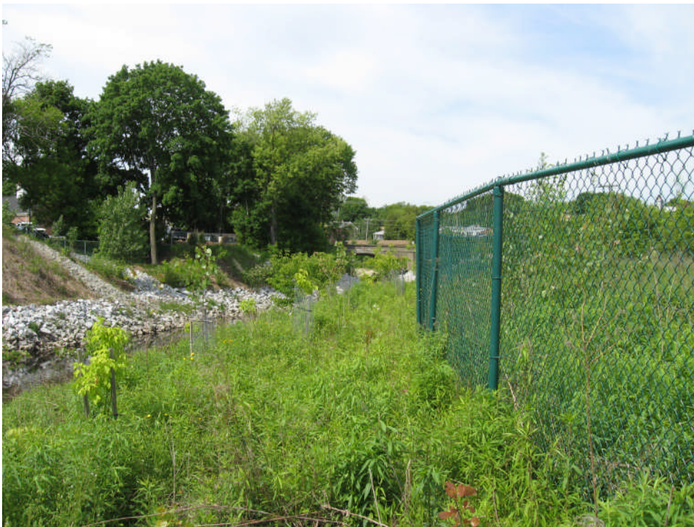
Photo 14: Upstream end of Planting Area #4, facing downstream (to the south/southwest).
