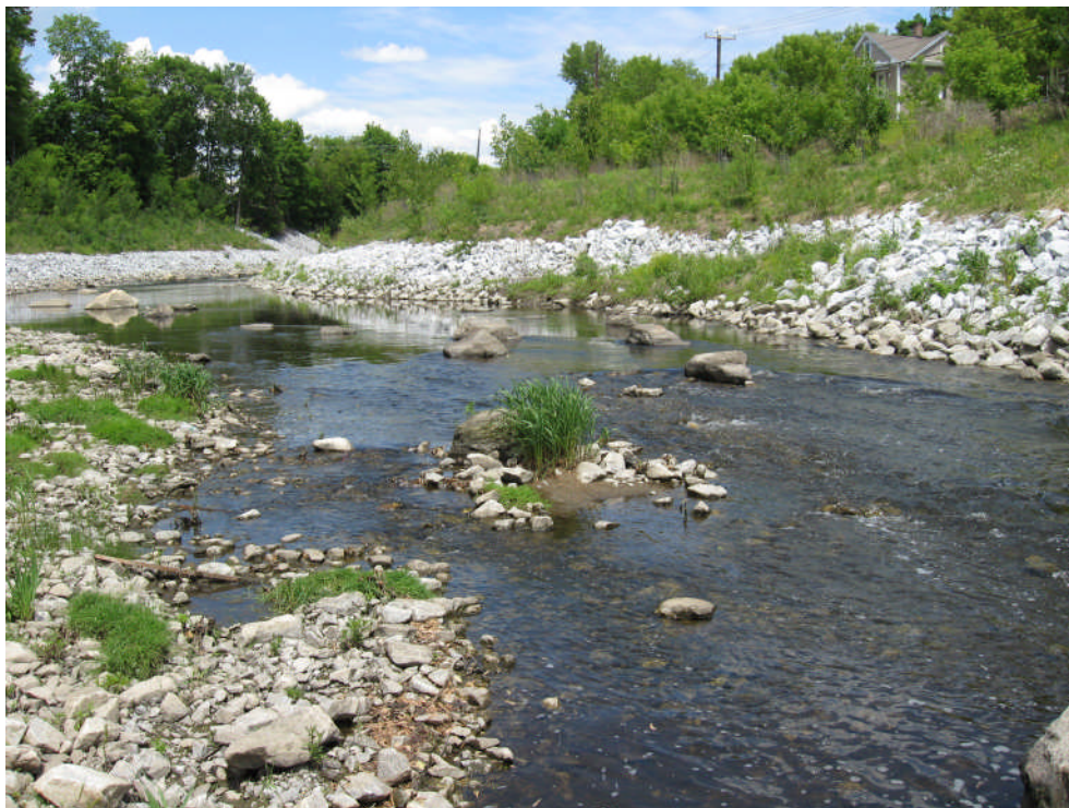
Photo 26: View of volunteer plants below the rip-rap line in the Phase 2 area.
