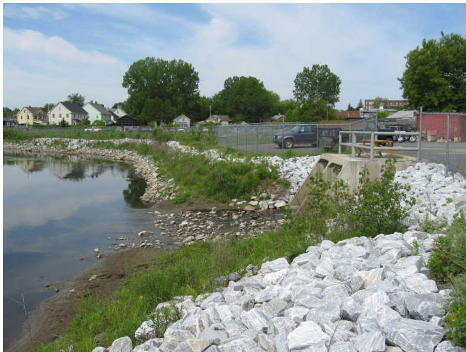
Photo 8: View of the twin box culverts that compose the New Silver Lake outfall, facing downstream (to the west).
