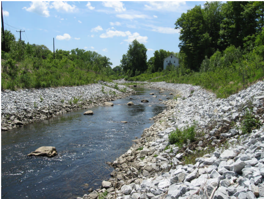
Photo 24: Alternate views of Planting Area #9 (right side of photo) and Planting Area #12 (left side of photo), facing downstream (to the southwest).
