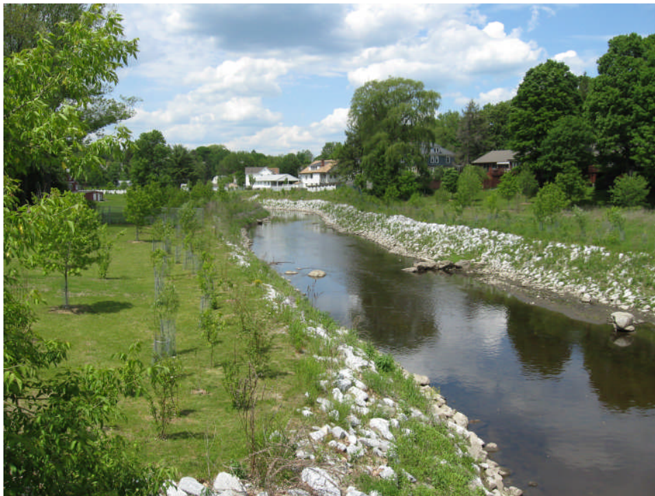
Photo 33: View of Planting Area #27 on the left side of the photo and Planting Area #38 and Monitoring Plot 3-E-3 on the right side of the photo, facing upstream (to the north/northeast).
