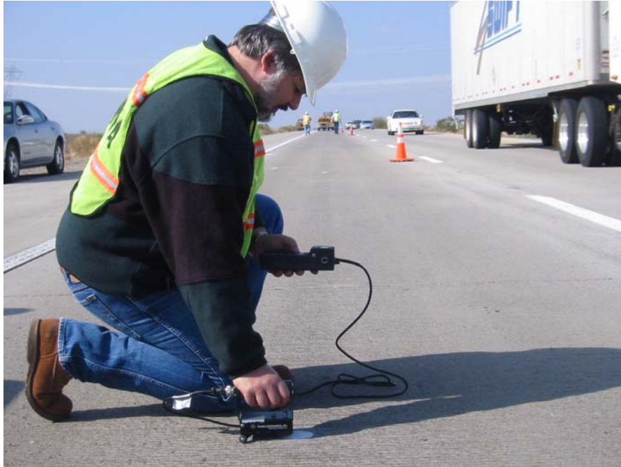
Figure 1. CTG-1 testing in progress.
