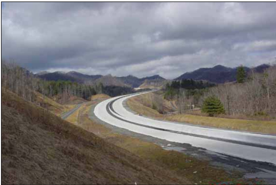
Figure 1. Completed concrete pavement on Future I-26, Madison Co., NC.
