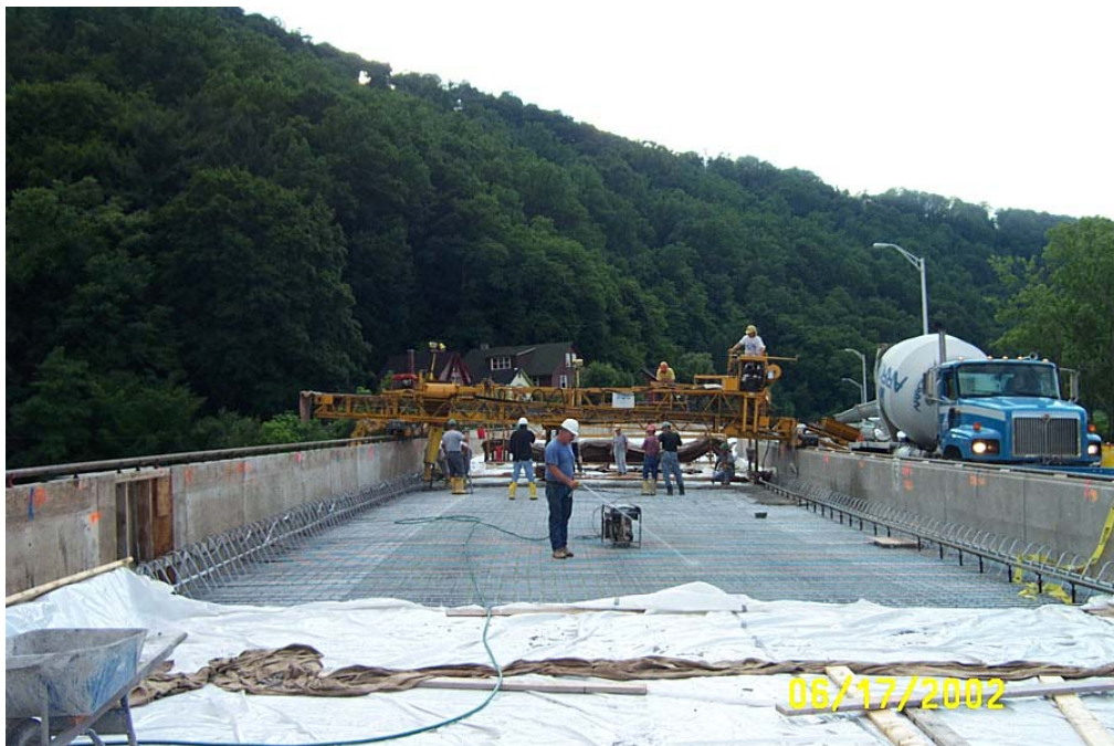
Figure 1: Concrete placement on the eastbound lanes
