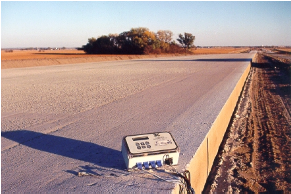
Figure 3. Pavement instrumented with maturity meter
