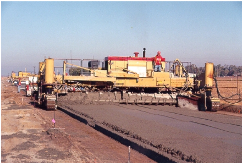
Figure 1: Concrete placement
