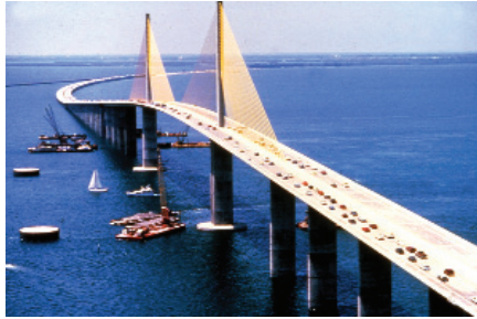
Figure 3-4. Fly ash concrete is used in severe exposure applications such as the decks and piers of Tampa Bay's Sunshine Skyway Bridge.
