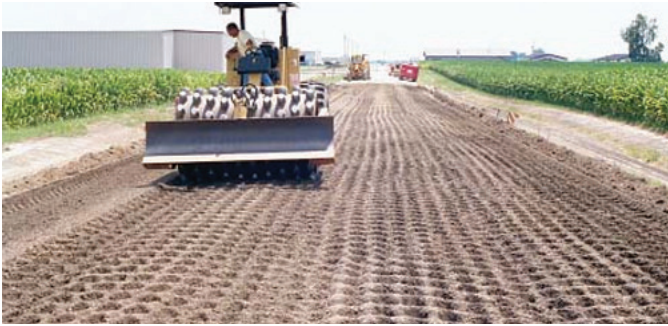
Figure 7-2. Compaction of fly ash stabilized soil.
