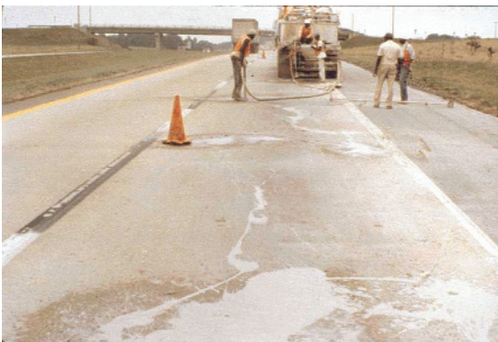
Figure 9-1. Fly ash grouts for pavement subsealing
