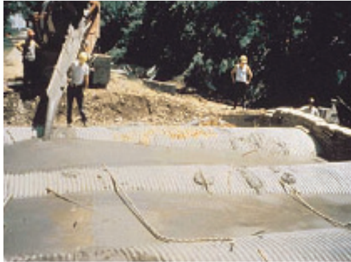
Figure 5-2. Flowable fill eliminates the need for manual compaction
