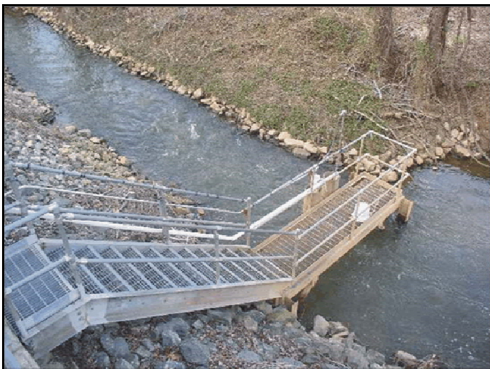
Figure 3-2. DuPont Spruance Final Outfall
