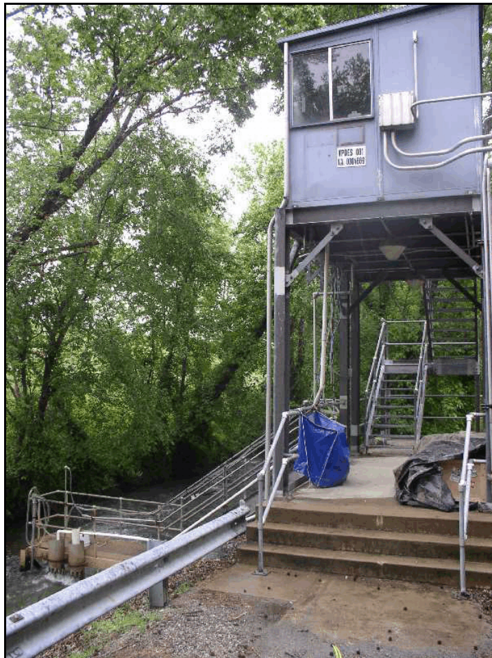
Figure 3-3. Test Site Showing Analyzer Shelter
