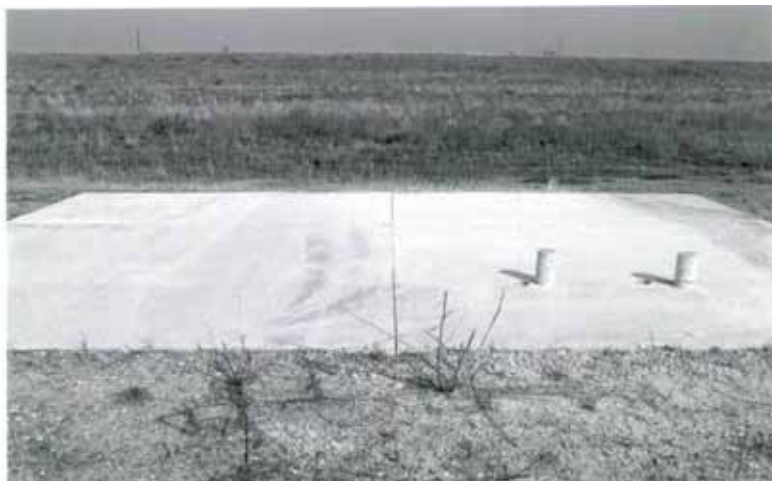
Figure 1. Test panels for mixture MN7 showing cores taken in 1994.
