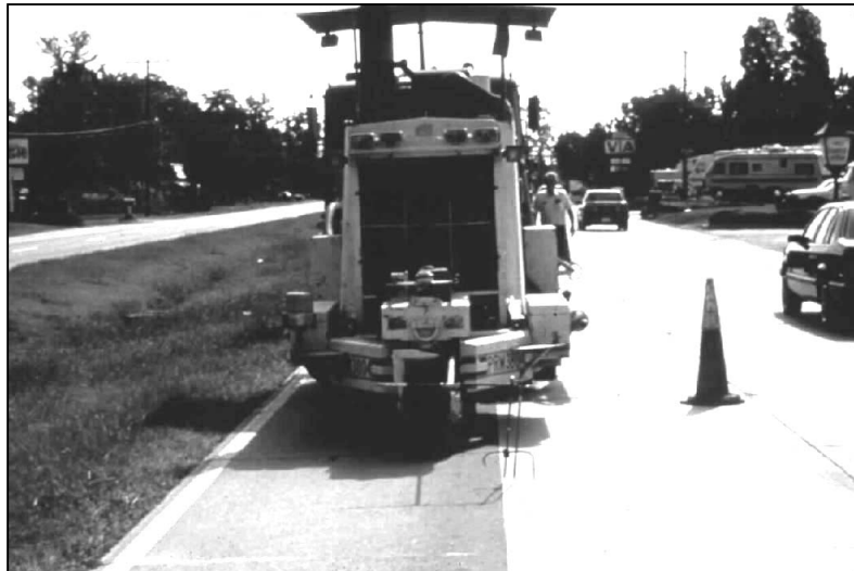
Figure 6. Diamond grinding equipment making multiple passes to grind a full lane width.
