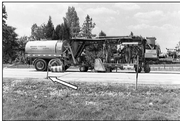
Figure 9. Slurry residue of diamond grinding being discharged to the embankment in a rural area.
