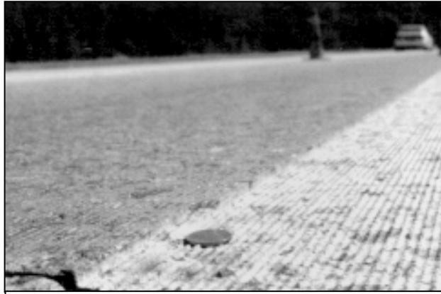
Figure 5. Final "corduroy" texture produced by diamond grinding.
