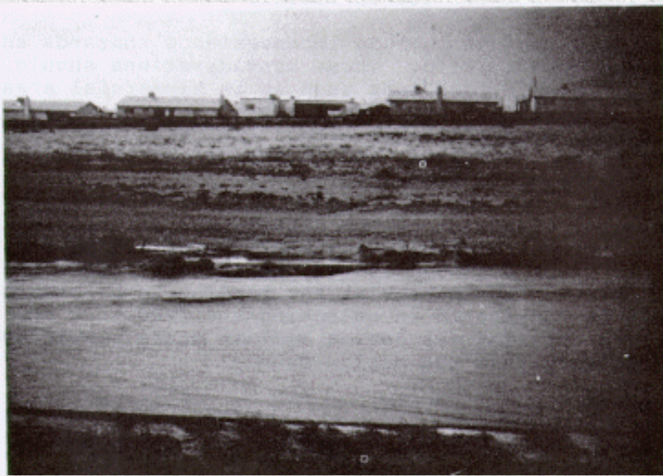
Figure 1. Spread greater than "allowable" spread on a major arterial.
