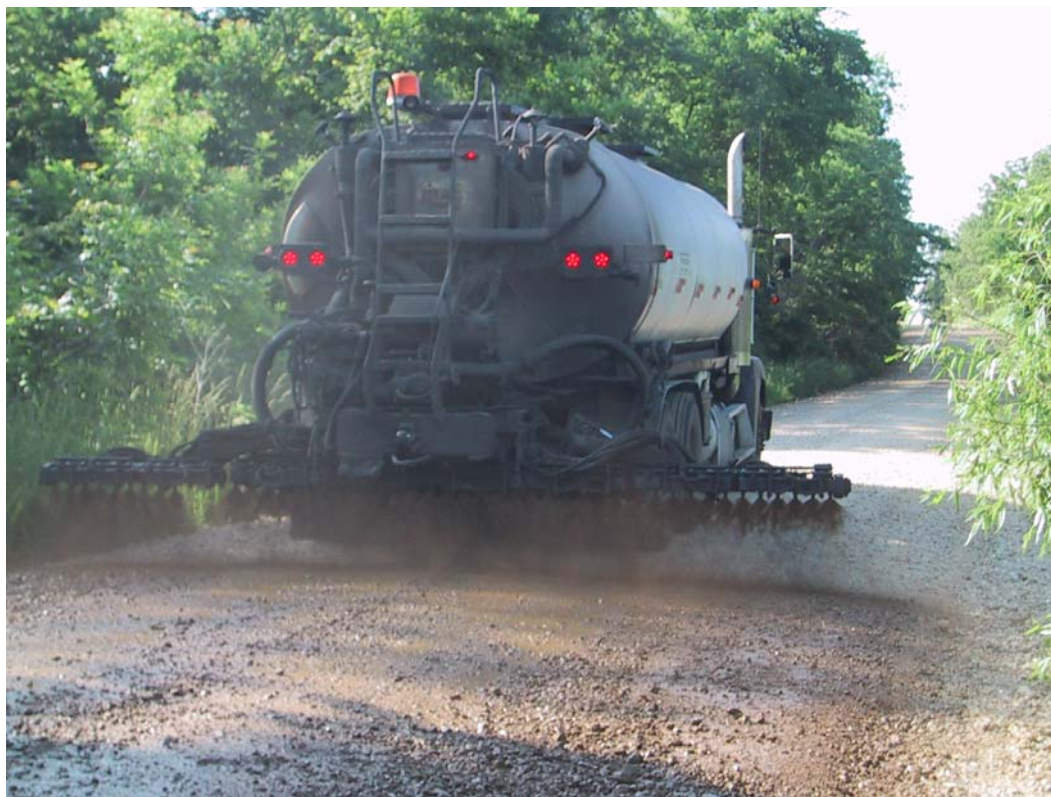
Figure 2. Application of PetroTac product at FLW
