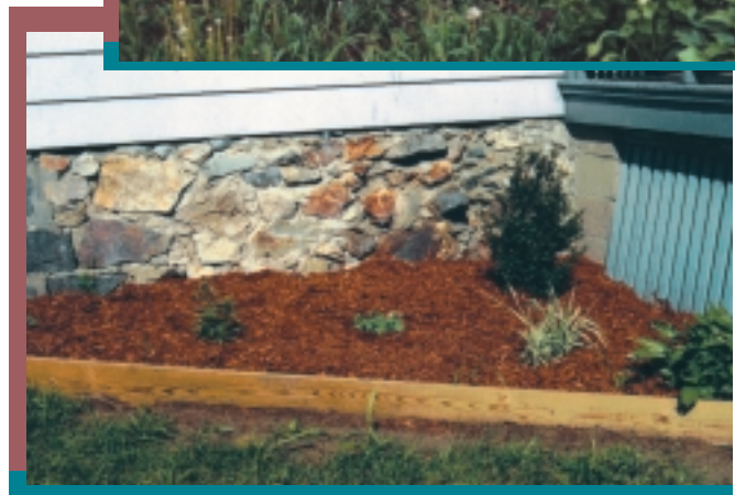
Top: Before—bare soil in drip zone (1660 ppm). Bottom: After—mulched planting bed covering soil.
