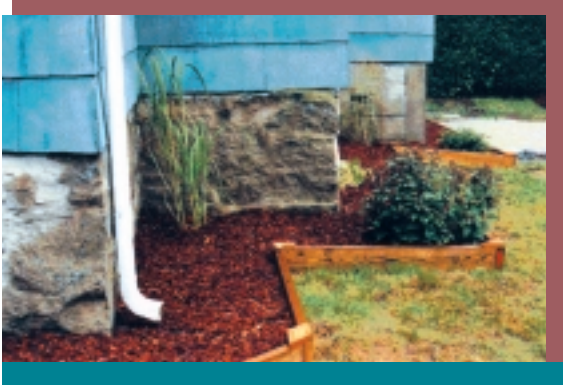
A perimeter mulch bed covering the drip zone.
