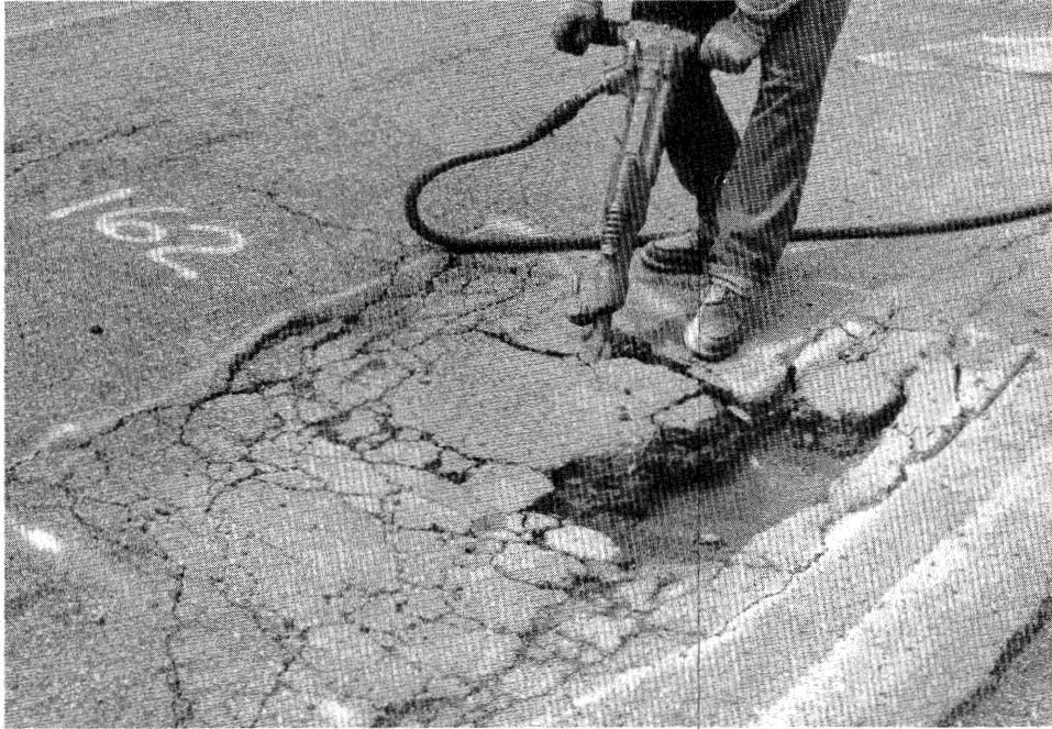
Figure 7. Cutting operation for standard procedure.
