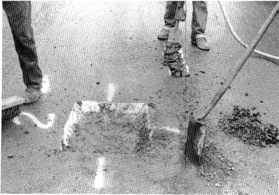
Figure 8. Cleaning operation for standard procedure.
