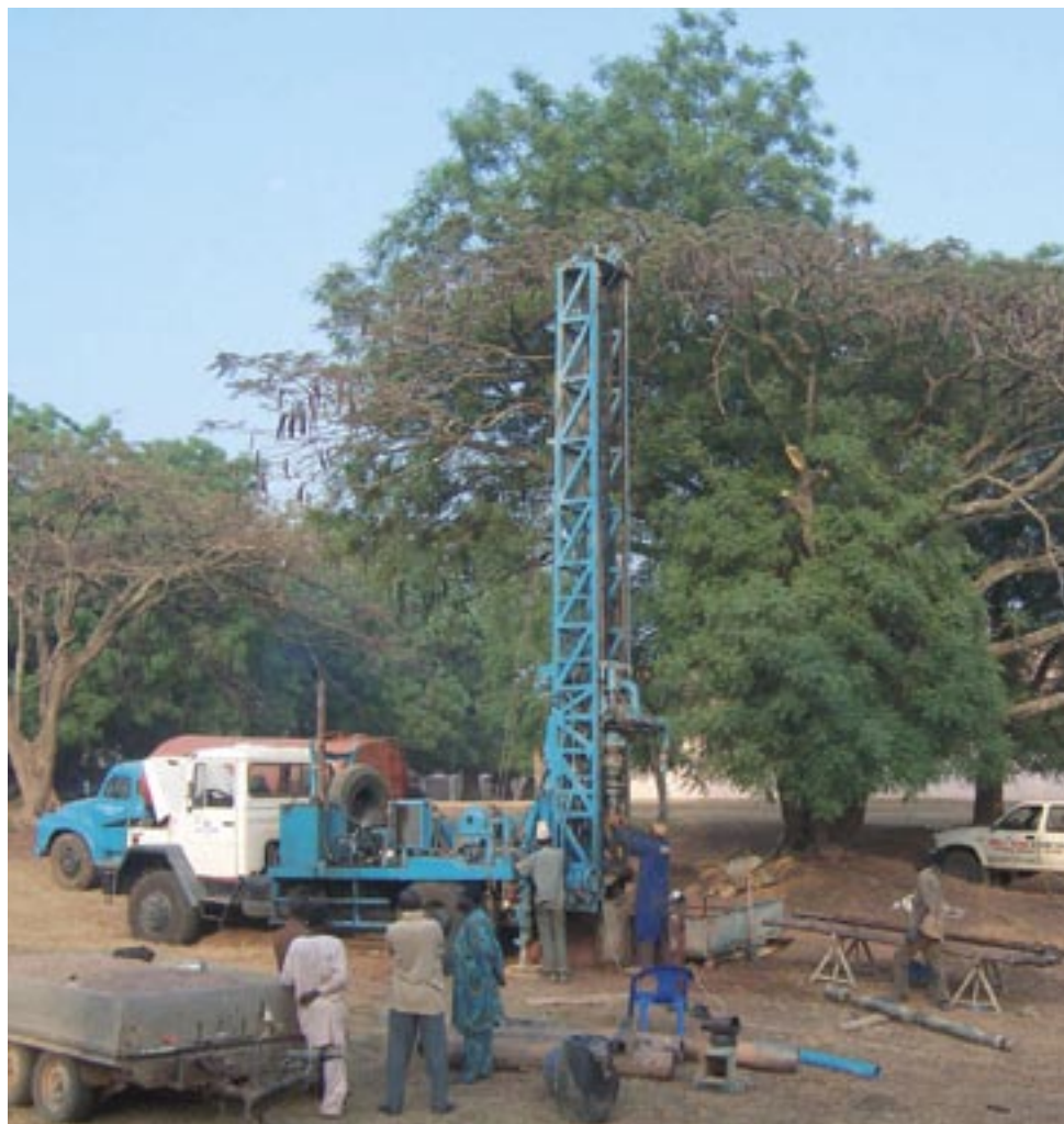
Workers build a water system for a Nigerian hospital with the help of a VfP volunteer.
