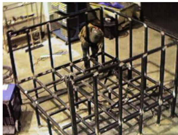
Figure 1. Photo. Culvert headbox under construction.
