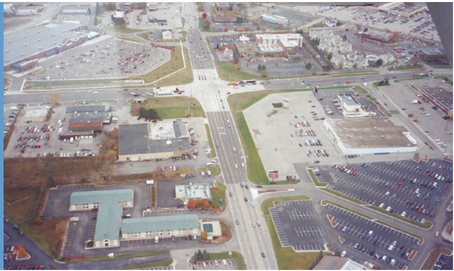
M-11 and M-37 Looking West (after)
