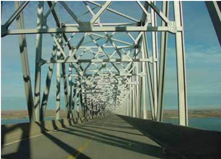
Forest City Bridge on US 212 over Lake Oahe, SD
