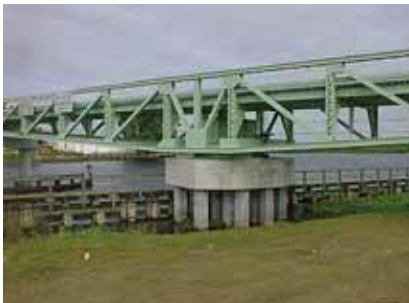
Lake Okeechobee Rim Canal Swing Bridge in Palm Beach County, FL
