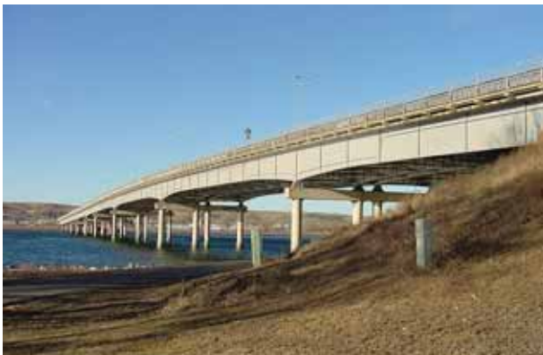
Fort Pierre Bridge on US 14 over the Missouri River, Pierre, SD
