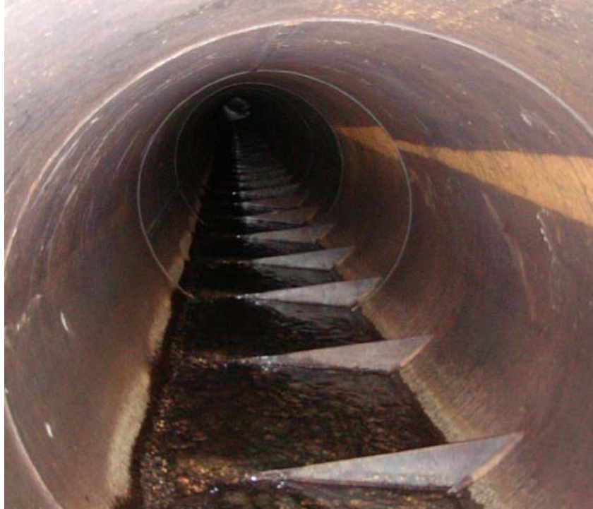
Figure 8.14 Steel corner baffles welded to the pipe and spaced 1.22 m (4 ft) apart, John Hatt Creek
