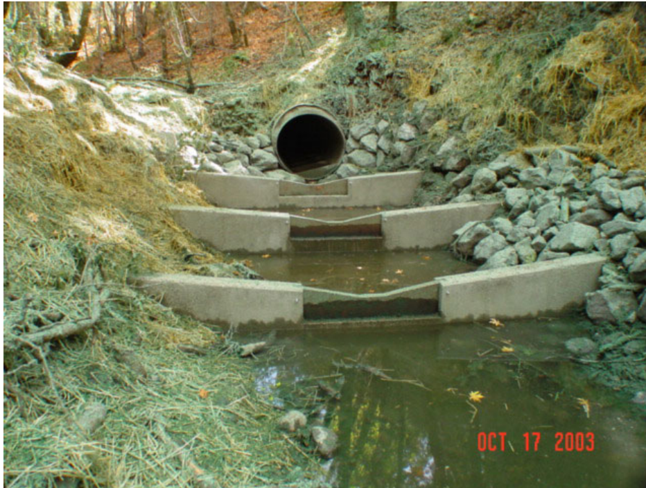
Figure 8.16 Culvert outlet after installation, John Hatt Creek
