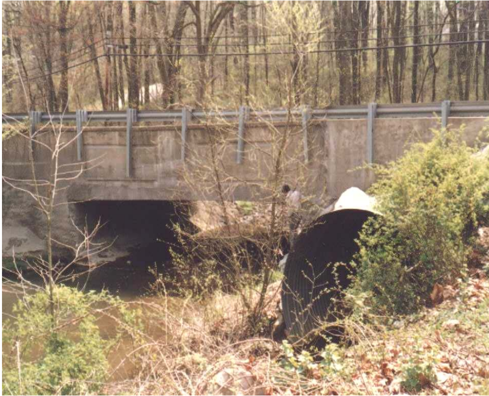
Figure 8.5 Pre-project channel condition (1992)
