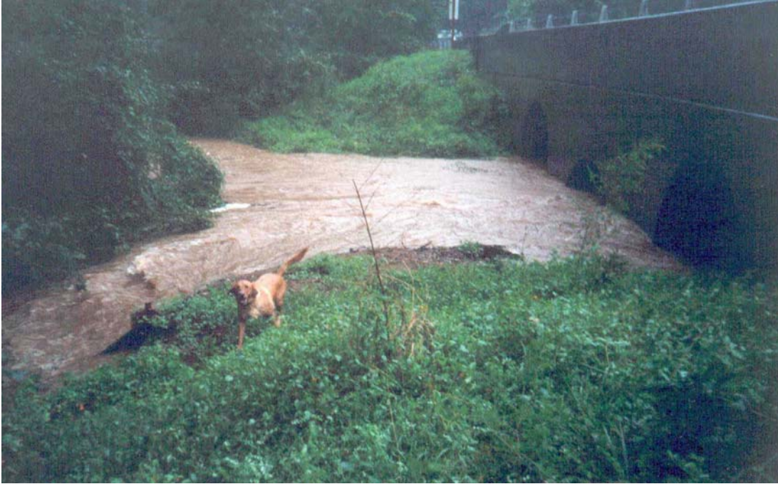
Figure 8.10 Upstream of current crossing during high-flow event
