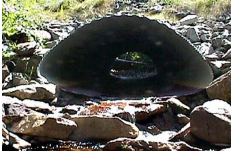
Figure 6.6 Downstream riprap will dissipate energy and reduce scour, but must be placed with fish utilization in mind (USFS 2005)
