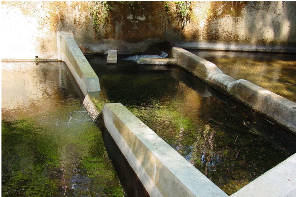
Figure 6.9 Notch weirs downstream of a culvert installation, acting to properly backwater the culvert, while maintaining manageable drops (United States Forest Service 2005)
