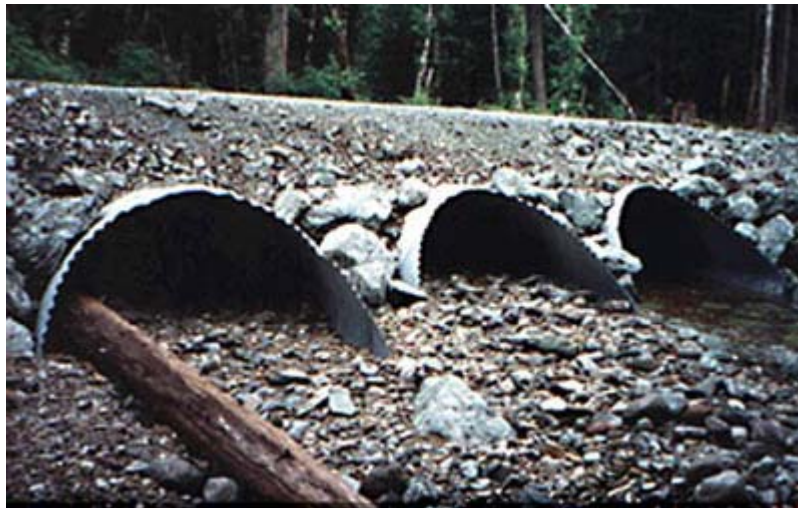
Figure 1.3 Multiple culvert installation located at a slope break where sediment is likely to deposit, creating a debris barrier (United States Forest Service 2006b)
