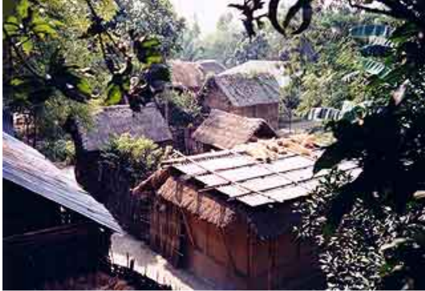
Figure 10. Photograph showing typical rural house in Bangladesh made of straw, mud, and timber frame
