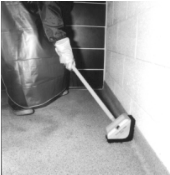
Use the corner brush to remove hard to reach debris. A coved corner helps in reducing the entrapment of dirt.
