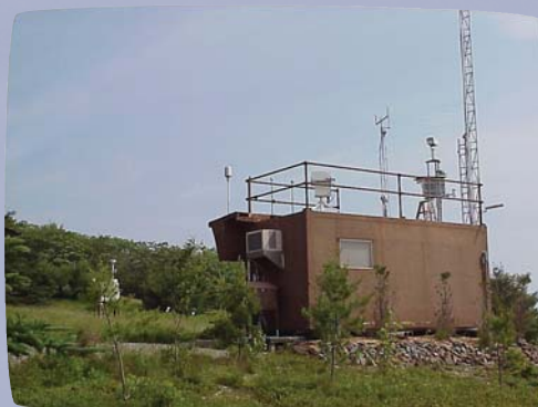
Air monitoring station
