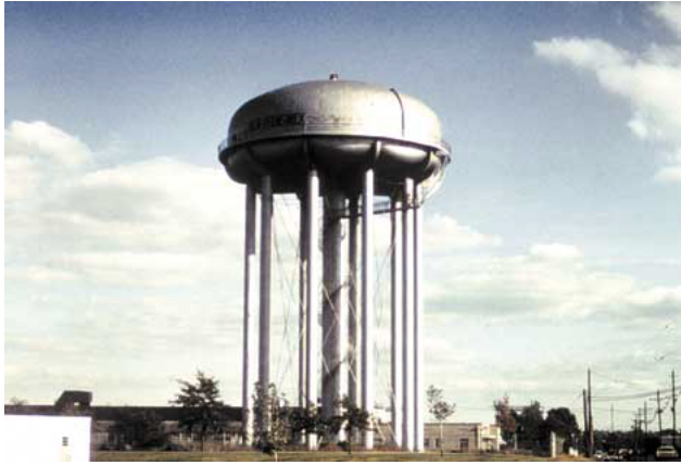
Water tower for public supply in central New Jersey. (Photograph by Eric Vowinkel)
