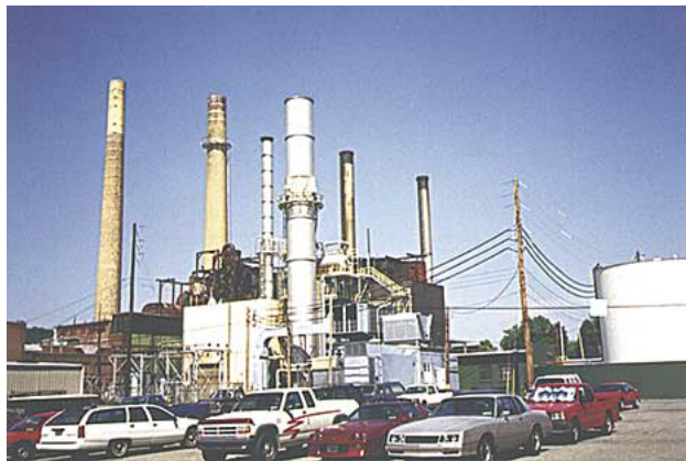
Industrial site, New Jersey. (Photograph by Rick Clawges)
