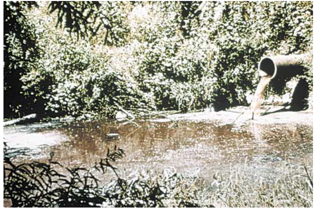
Wastewater discharge to stream. (Photograph by Eric Vowinkel)
