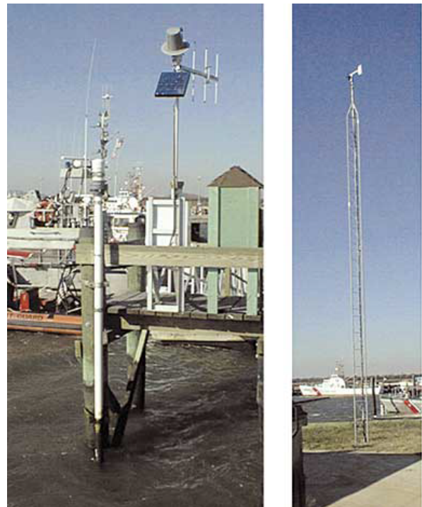
Tide-telemetry (left) and weather-monitoring equipment at Cape May Harbor at U.S. Coast Guard Training Center, Cape May, New Jersey. (Photograph by John Stepnowski, National Ocean Service)
