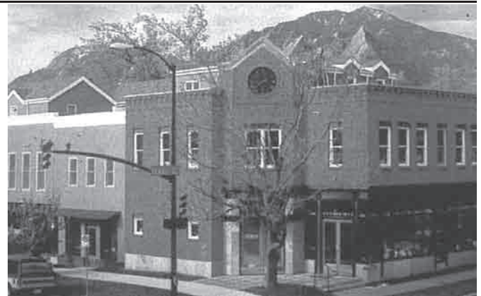
Active Commercial / Mixed Use Streetscape
