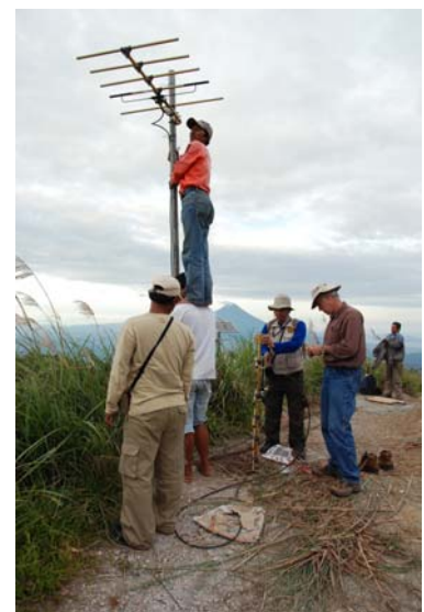
VDAP and CVGHM scientists install a station for sending data about volcanic activity in North Sulawesi. Courtesy of VDAP.
