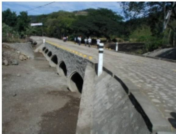
Figure 3. View of newly constructed El Hatillo bridge in Nicaragua
