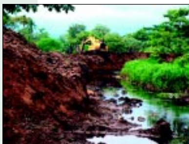
Structural mitigation project. Building a levee. Providencia, Guatemala
