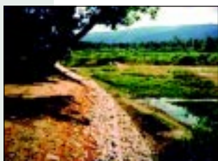
Structural mitigation project. Placing gabions. Jacmel, Haiti
