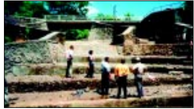
Structural mitigation project. Placing gabions below a bridge. Chichigalpa, Nicaragua
