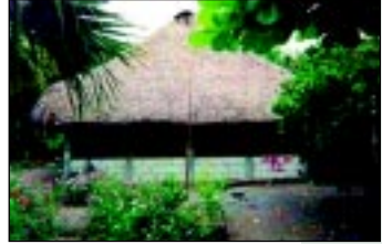
Non-structural mitigation. Floodwall around a house. Chiquimulilla Canal, Guatemala
