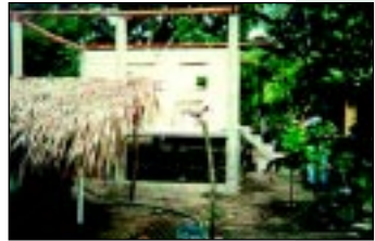
Non-structural mitigation project. Elevating a house. Chiquimulilla Canal, Guatemala
