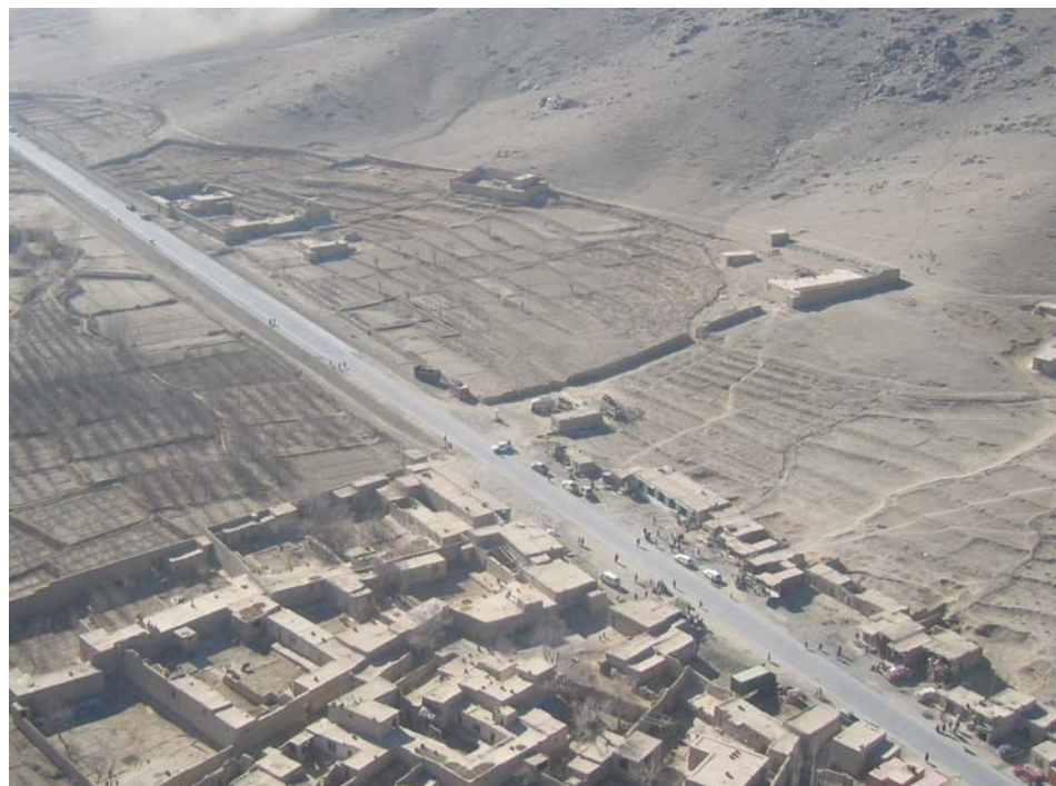
The rebuilding of the badly damaged 389-kilometer highway from Kabul, Afghanistan, to Kandahar was completed by USAID in December.
