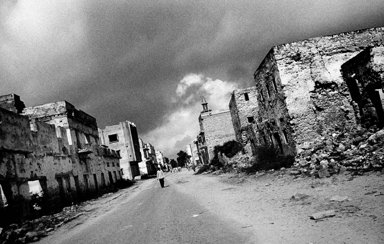
Destroyed buildings in Mogadishu, Somalia.
