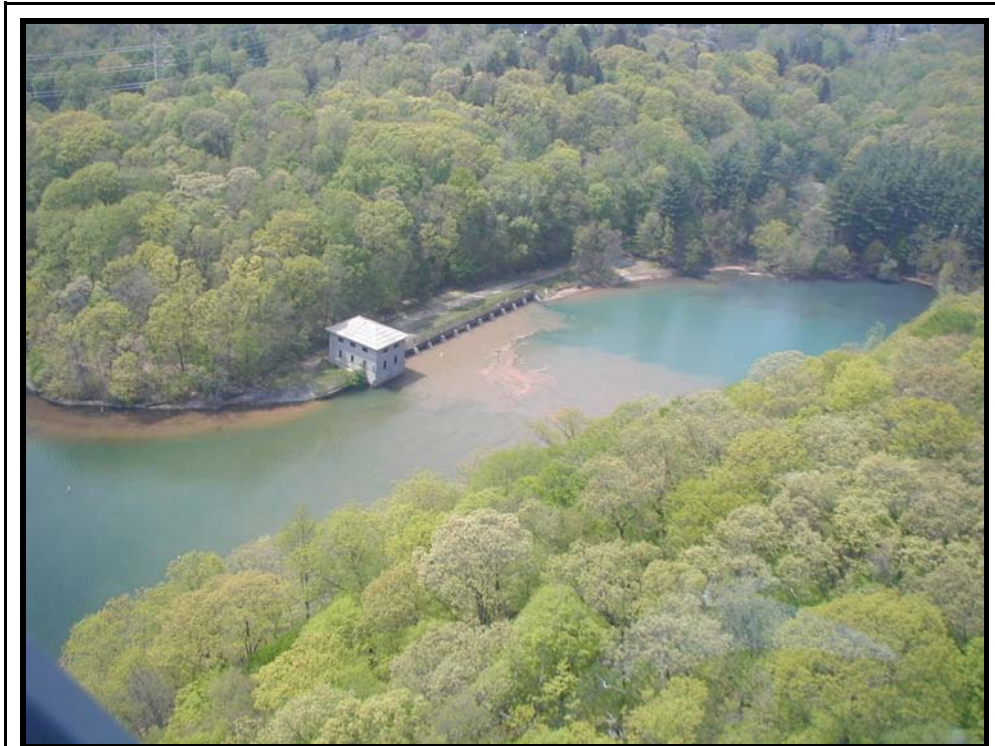
Figure 1.7 Photograph of the Catskill Influent Chamber Cove on Kensico Reservoir taken in May 2005 during alum treatment (looking approximately northwest).
