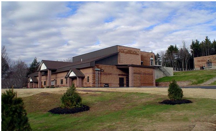
Figure 1.12 This wastewater treatment plant serving the Village of Hunter was constructed with funding from the City under the auspices of the New Infrastructure Program.
