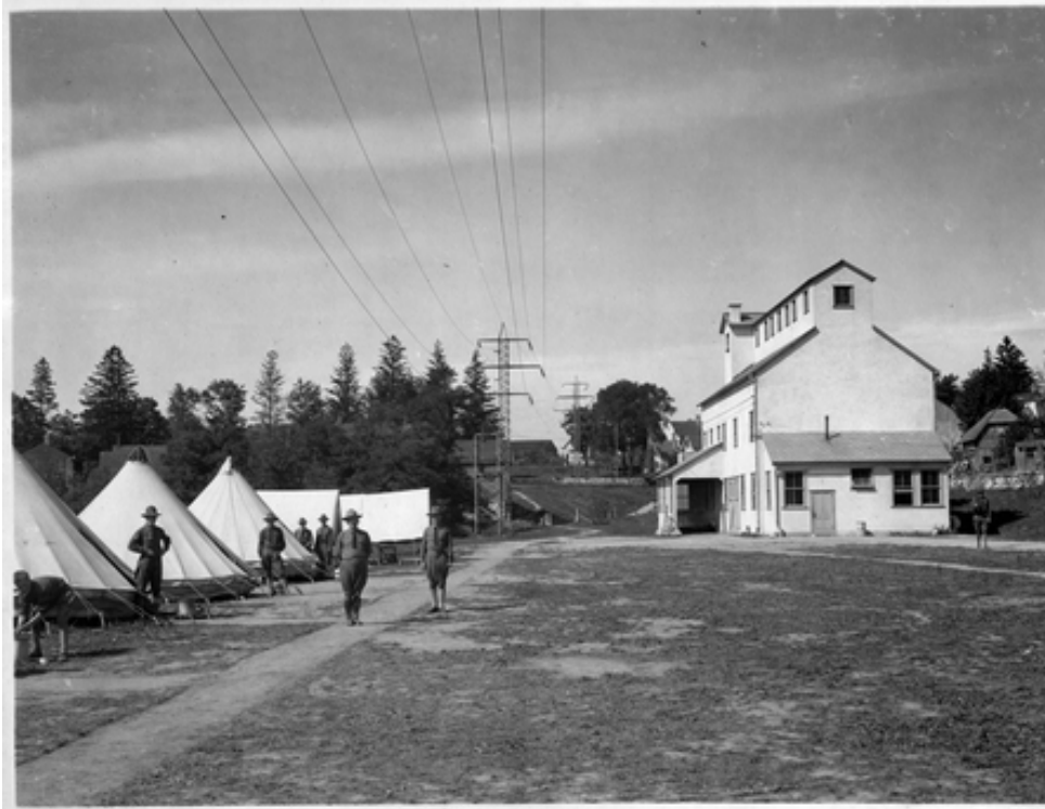
Figure 1.6 This picture of New York City's Board of Water Supply coagulating plant, taken September 19, 1917, indicates that turbidity was an anticipated water quality concern.
