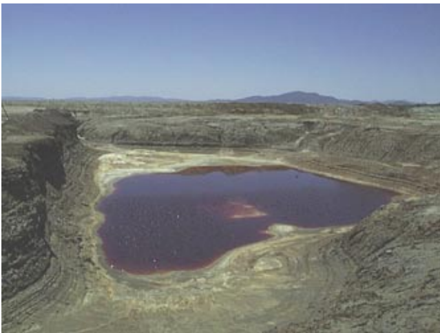
Photograph 11. A trench in the large tailings impoundment at Caselton collects and retains surface runoff. The sulfidic tailings create acidic, metal-rich waters that are further enriched by cycles of evaporation. Native sulfur crusts on the surface are a reactive source of sulfuric acid.
