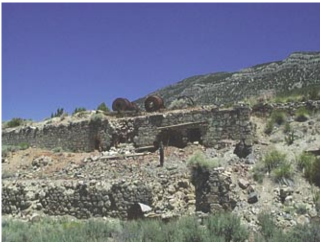
Photograph 2. This mill at Cortez is typical of older mills with its stone foundation and three levels. Newer mills in the 20th century were made with concrete foundations, and many had four to six levels.
