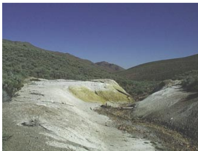
Photograph 7. Tailings from the Hilltop mill were placed in the canyon across from the mill with no regard for the small creek, which has eroded through the dam. This was standard practice through 1935, when the first regulations were established for tailings disposal.
