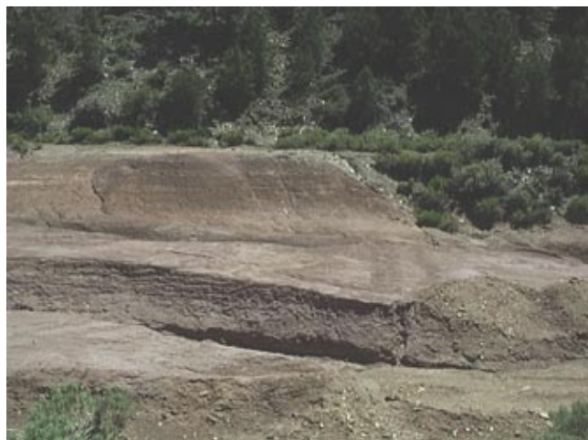
Photograph 10. This was one of the smaller tailings ponds below the White Caps mill at Manhattan. The dam, about 3 m high, was breached and most of the tailings eroded in one or more storm events.
