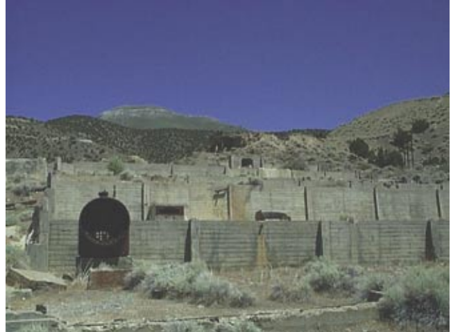
Photograph 3. This mill at Lower Rochester operated from 1913 to 1929 at about 150–300 tons/day. This relatively large mill utilized the best cyanide technology of the time. Concrete was used in foundations after about 1900.
