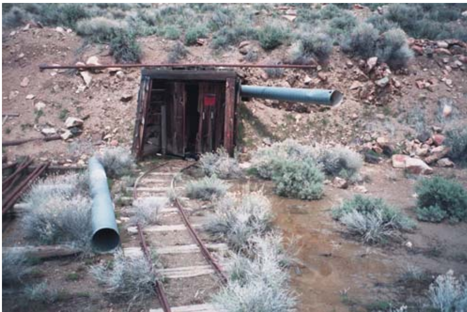
Photograph 2. The Majuba mine adit releases a small amount of water with a pH of 7.4 and low metal concentrations. It is not a problem.
