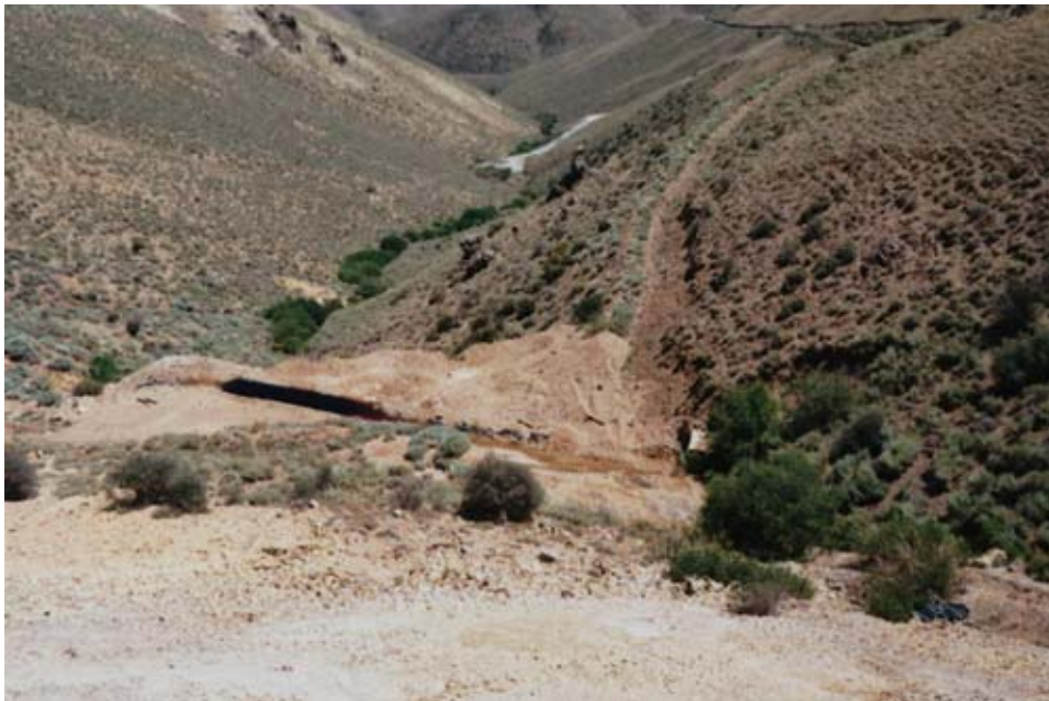
Photograph 12. A series of mine tunnels in the Dean Mine complex released acidic drainage that reacted with sulfidic waste rocks. The siliceous wallrocks at the upper tunnels provided no acid neutralization, but the lower tunnel (gray rocks, upper part of photograph) was in limestone and the mine drainage was near neutral. These tunnels were plugged and the dumps reclaimed in 1998, with major improvements in water quality.
