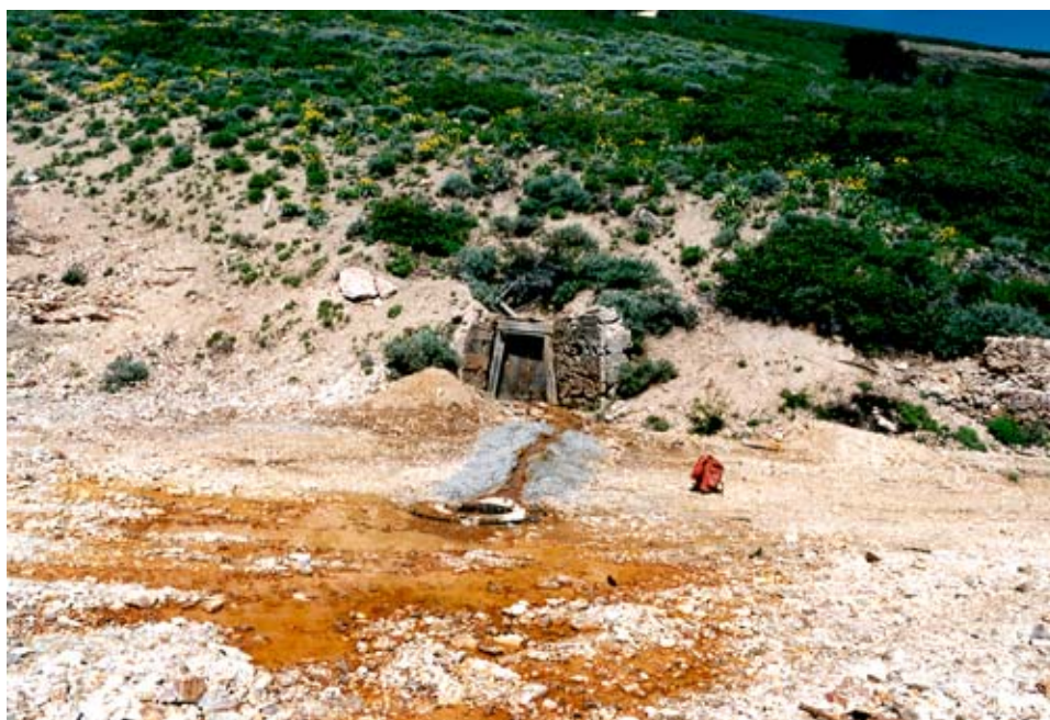
Photograph 1. The Buckskin National mine tunnel releases a moderate flow of water during spring snow melt. Reclamation in about 1997 created the cement trough and underground drain to minimize reactions with the mine waste dump. The pH is 3.0.
