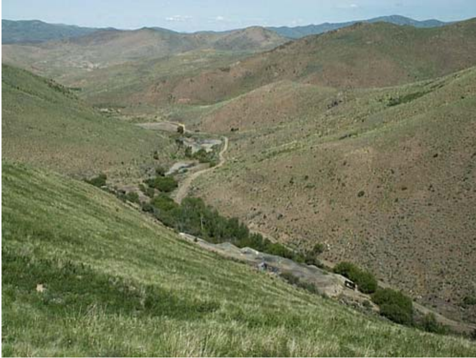
Photograph 16. View of Rip Van Winkle mine area with tailings six ponds in Coon Creek. The mine tunnel and waste dump (dark gray) are in the right side of the view.
