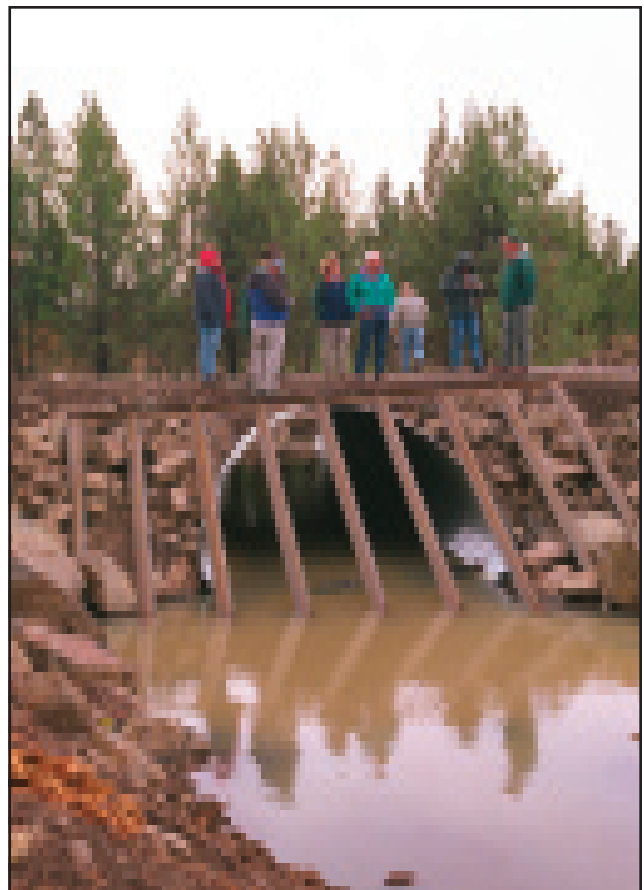
Debris racks at culvert inlets can prevent clogging.
