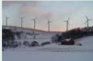
Exelon Community Energy Wind Farm at Mill Run
