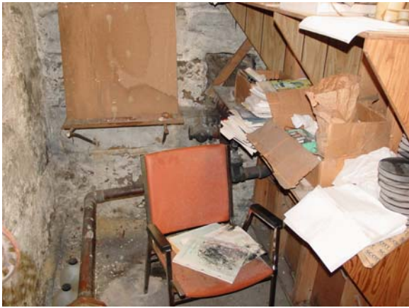
Figure 29. District Attorney's storage area in basement.
