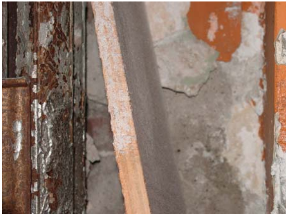
Figure 25. Cabinet in front office of the Clerk of Courts.
