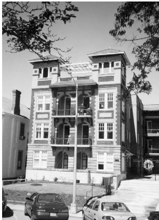
Katherine 6.2: A major work item in the Katherine Court rehabilitation project was the reconstruction of the building's missing towers. These features fully recapture the building's Renaissance Revival appearance.
