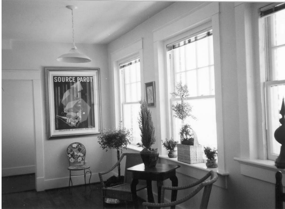
Katherine 6.3: Repairs to the Katherine Court Apartments such as windows, window trim and wood floors, allowed the apartments to retain their historic character and materials.
