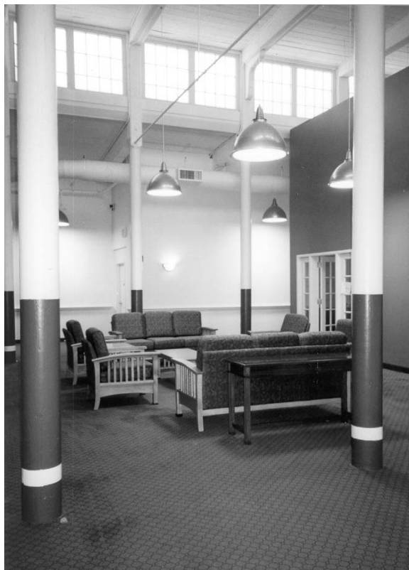
Whitman 6.8: A community seating area exhibits the mill's historic character in its exposed historic posts and beams, as well as large clerestory windows.
