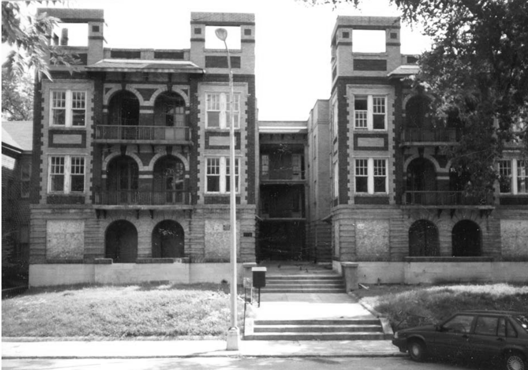
Katherine 6.1: Boarded and neglected, the Katherine Court Apartments were vacant prior to the rehabilitation.
